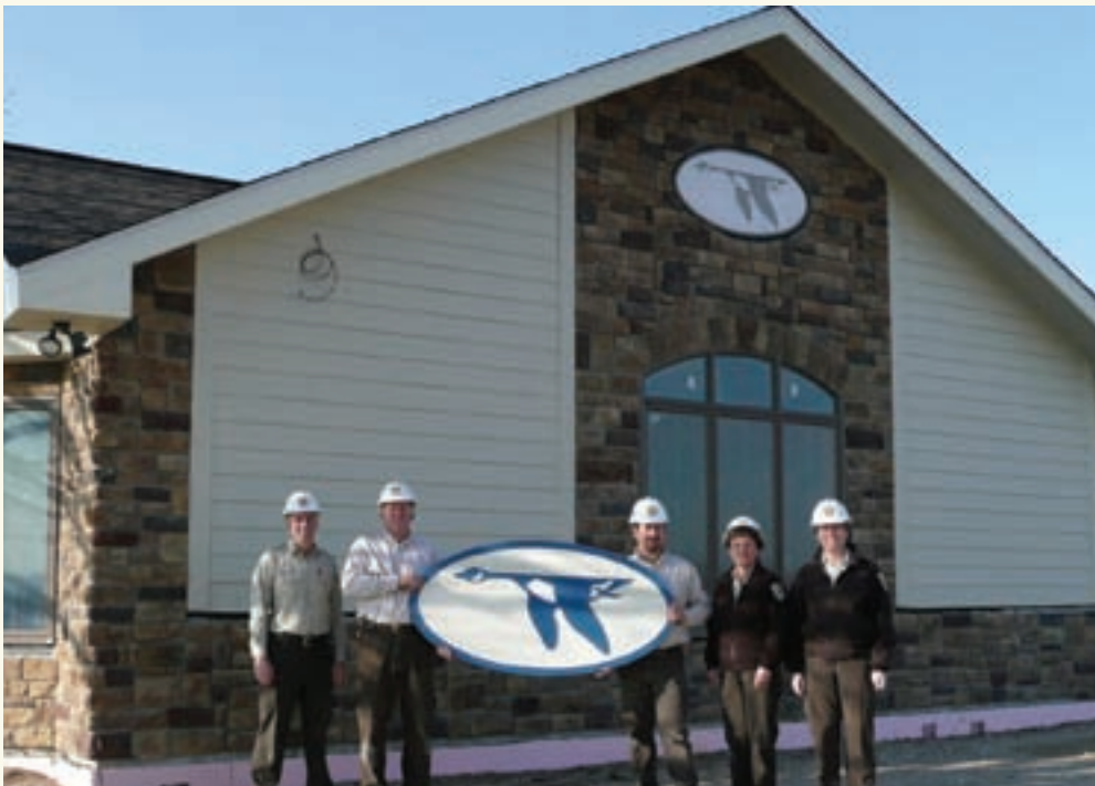
A Midwest Region Maintenance Action Team completed its most ambitious assignment to date – renovating and expanding the 35-year-old headquarters building at Clarence Cannon Refuge in Missouri. Holding the Blue Goose high are refuge employees (left to right) refuge manager Dave Ellis, maintenance mechanic Alan Lagemann, maintenance worker Kurtis Pursley, administrative technician Carolyn Gregory, and wildlife specialist Candy Chambers. (USFWS)
