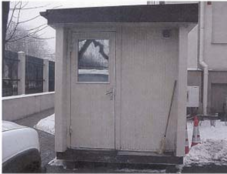
Figure 9: Inadequate Compound Access Control Booth
