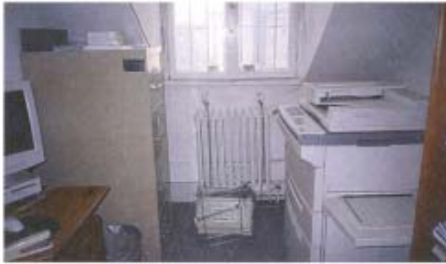
Figure 11: Chain-link Ladder Serves as Fire Escape for 6 th Floor Embassy Employees
