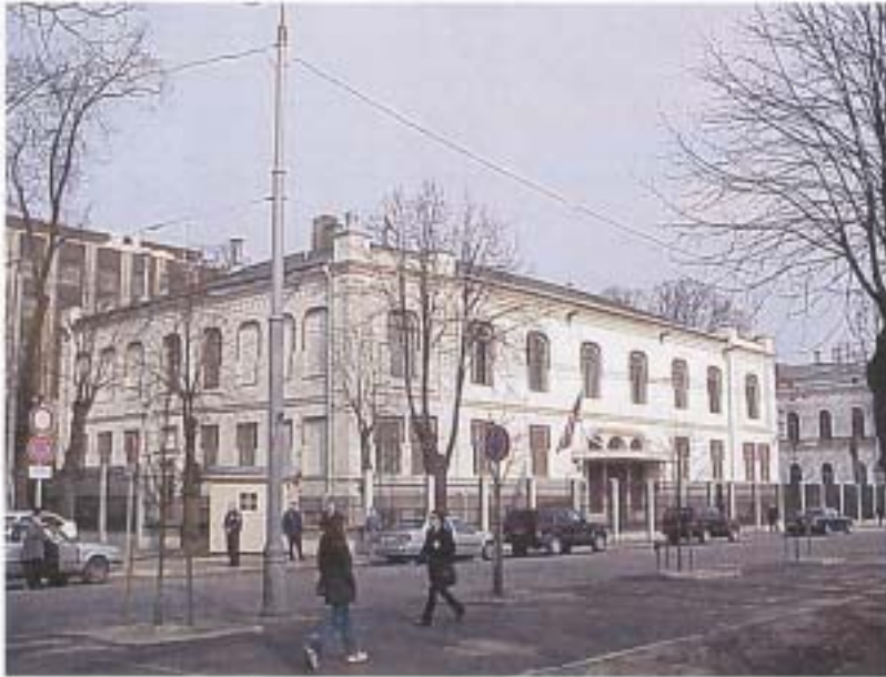
Figure 6: Insufficient Setback at a U.S. Embassy
