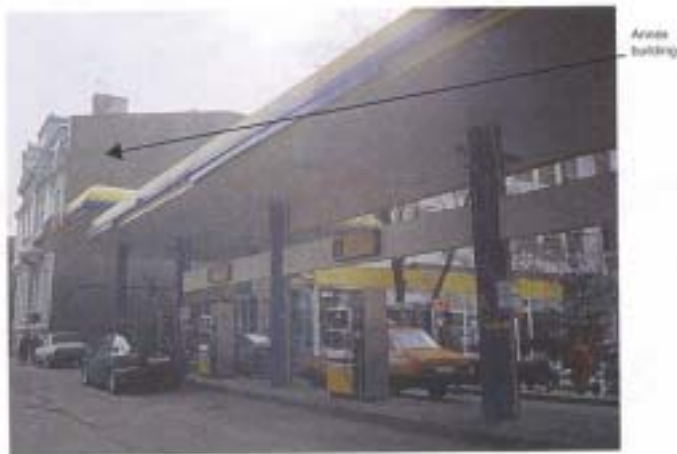
Figure 7: Public Gas Station Behind an Embassy Building Poses Security Concern
