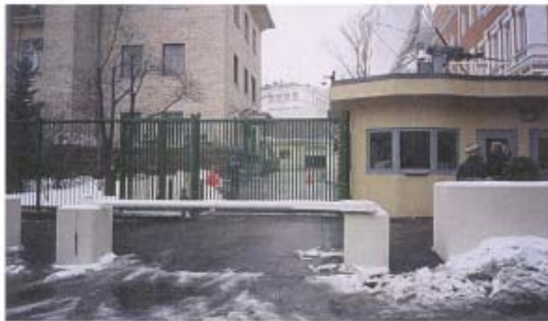
Figure 10: Newly Upgraded Compound Access Control Booth
