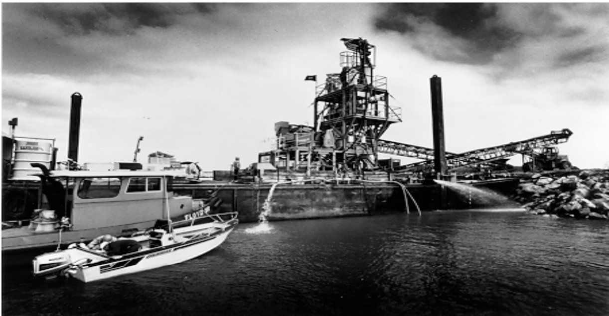
Bergmann Soil and Sediment Washing
