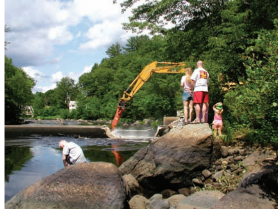
The Henniker dam during removal.
