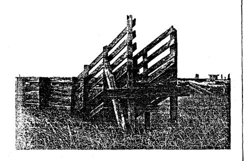
Note the random construction (varied board widths and lengths) and high level of deterioration due to fungal attack and corrosion of nails.
