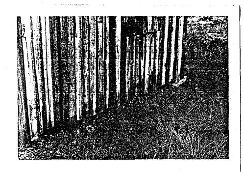
Wood rotted pilings, boards, and batts is a problem with both bunkhouses.
