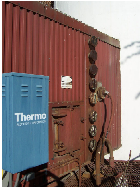
Figure 2-2. Test Port Locations for Boiler 10
