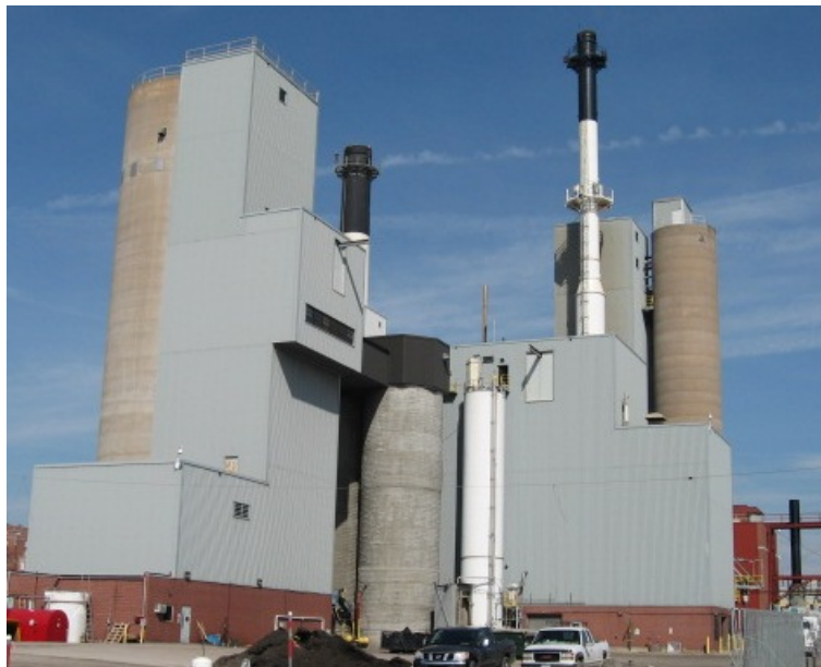
Figure 2-1. The University of Iowa Main Power Plant
