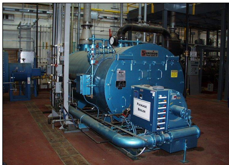
Figure 3-1. Wetback Scotch Marine Package Boiler
