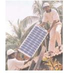
bank loans for financing sales of SELCO's solar home systems to Sri Lankans, through a local nonprofit microfinancing institution. SELCO's solar systems, which sell for between \$450 and \$650, convert sunlight directly into electricity through roof- or pole-mounted solar photovoltaic modules, which charge deepcycle batteries with DC current. The modules can produce power for up to 25 years, and are guaranteed by SELCO for a minimum of ten years.
