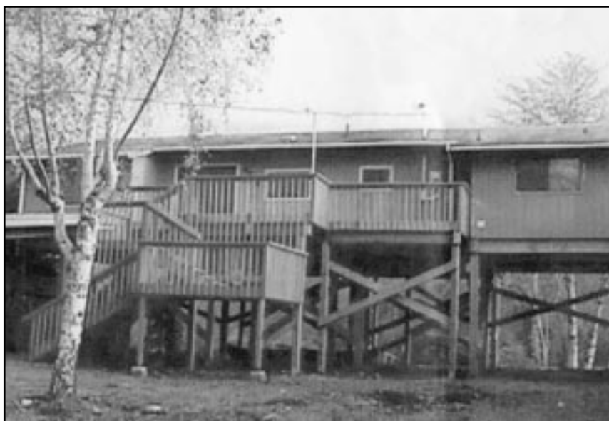
Home in Oregon elevated with FMA/ICC funds.
