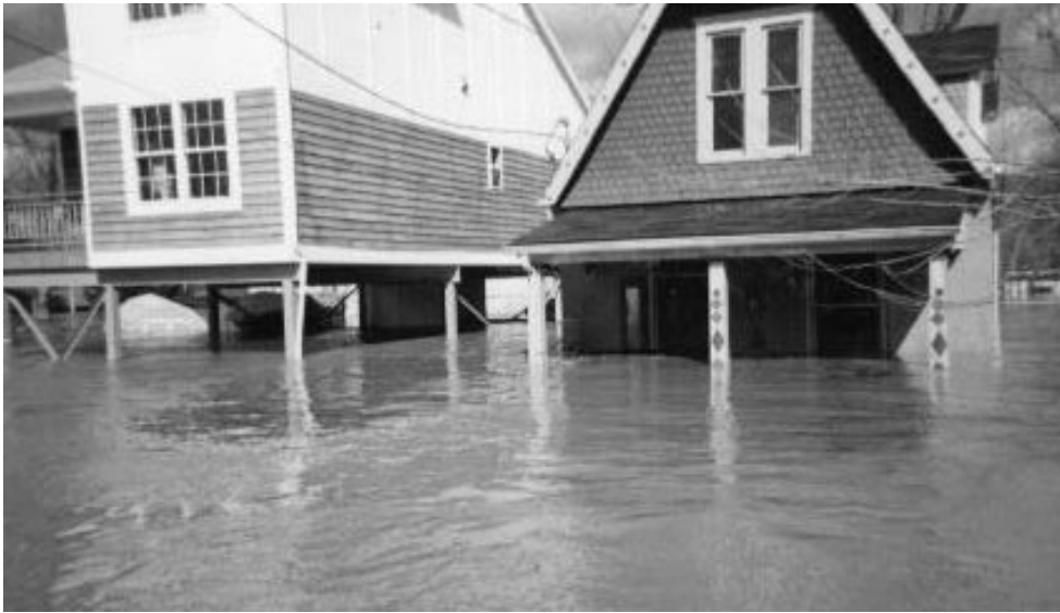
As floodwaters receded, the elevated house on the left suffered less damage than neighboring ones.
