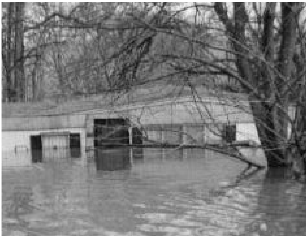
Some simple actions can protect homes, such as this mobile home, from future flood damage.
