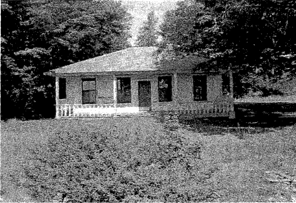
Figure 4.117. Frederick H. and Mary Trude cottage, front (eastern) elevation, 1996. The Trude cottage is one of three Cottage Row houses that appear to be influenced by vernacular dog-trot bungalows, a common house type in Gulf Coast resort communities. The broad front gallery of the Trude cottage takes advantage of the building's orientation toward the Manitou Passage.
