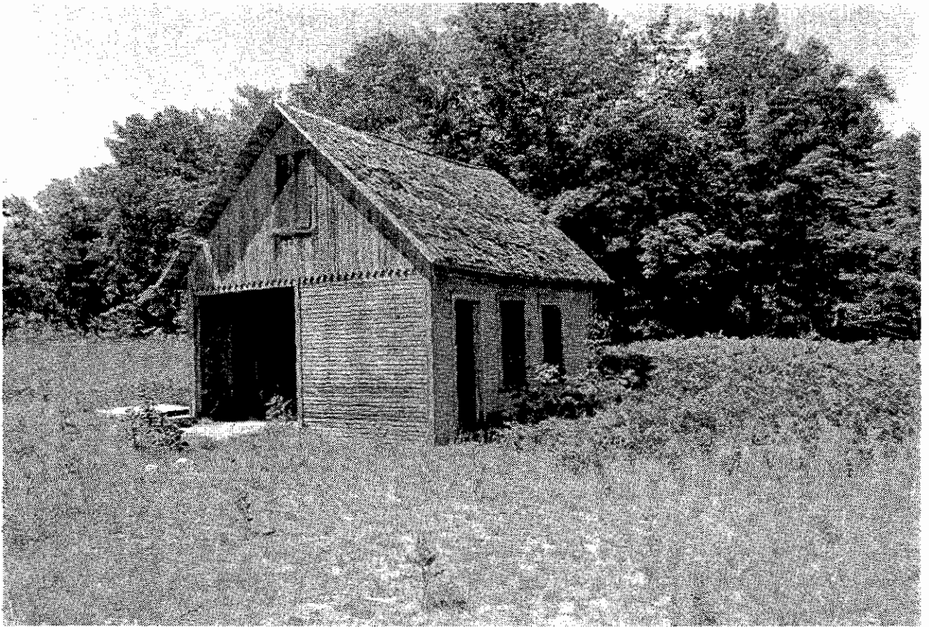
Figure 4.58. Alvar and Mary Bournique automobile garage, 1996. The Bourniques probably found their automobile to be a convenient and efficient mode of transportation from their remote summer home at the southeastern tip of the island. However, the difficulty of maneuvering early-model automobiles over the property's loose, sandy soils is suggested by the remnant corduroy driveway that extends outward from the western garage entrance. Other segments of corduroy surface may remain elsewhere on the Bournique farm, buried beneath drifts of sand.
