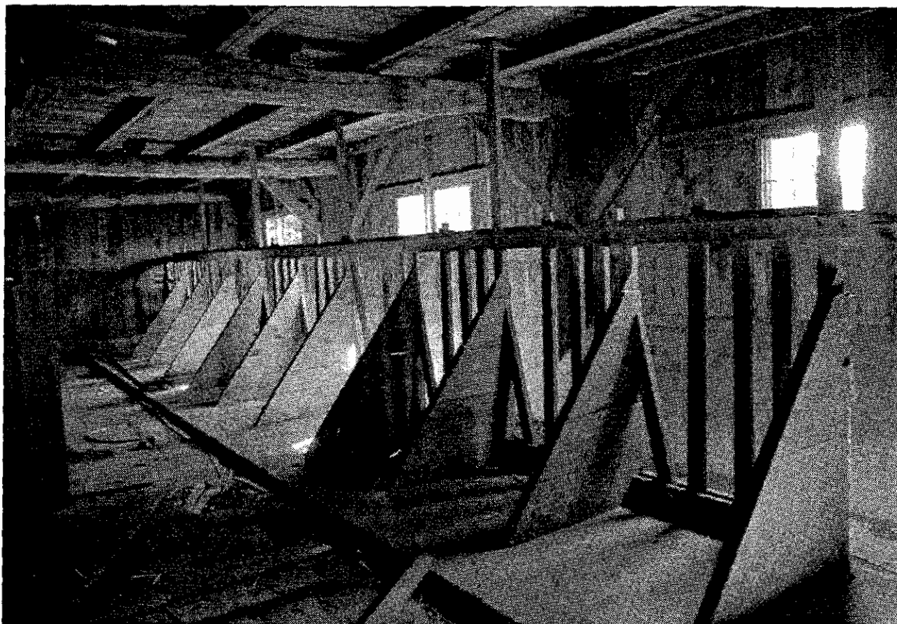
Figure 4.37. Manitou Island Association west-side barn, milking stanchions, 1996. The floor plan, materials, equipment, and interior finishes of the MIA barn conform to standards promulgated during the 1910s and 1920s by the U.S. Department of Agriculture and the extension programs of state agricultural colleges.
