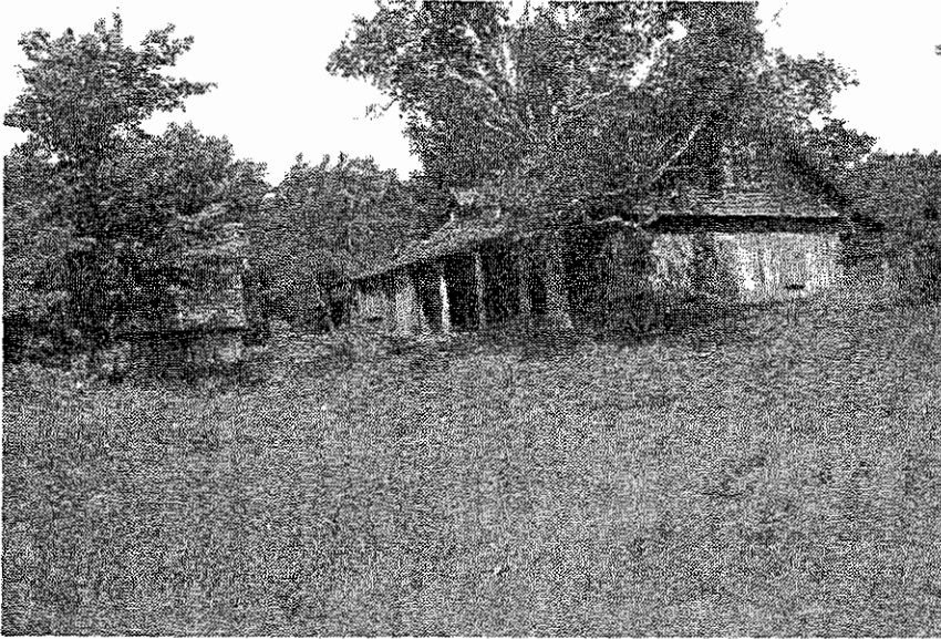
Figure 5.23. Alvar and Mary Bournique residence and ice house, 1996. The complex retains historical integrity, but it is deteriorating rapidly.
