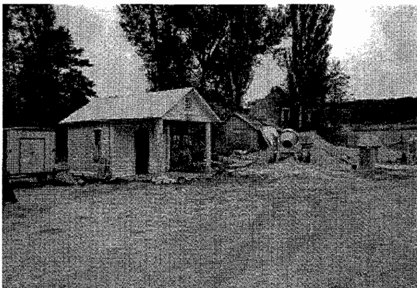
Figure 4.17. Manitou Island Association gas station. A small gas station stands opposite the equipment shed, along the southern edge of the farm yard. The gas station represents a specialized building type—one made necessary by the MIA's utilization of large machinery powered by fossil fuels. Along with the equipment shed, the gas station is a key resource in distinguishing the MIA farm as a modern, "neotechnic" agricultural enterprise.
