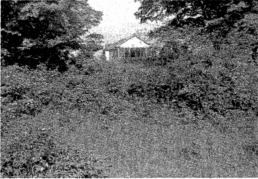
Figure 4.122. Howard W. Foote cottage, 1996. Like other Cottage Row houses, the Foote cottage originally fronted onto a boardwalk that extended along the edge of the beach ridge.
