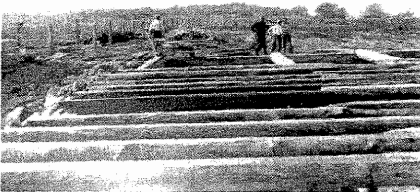
Figure 4.5. Manitou Island Association barn during construction, 1927. The large, modern, gambrel-roofed barn was the centerpiece of the MIA's farmstead at North Manitou Village. It was built on a site amidst the farm formerly operated by Silas Boardman and the Newhalls.
