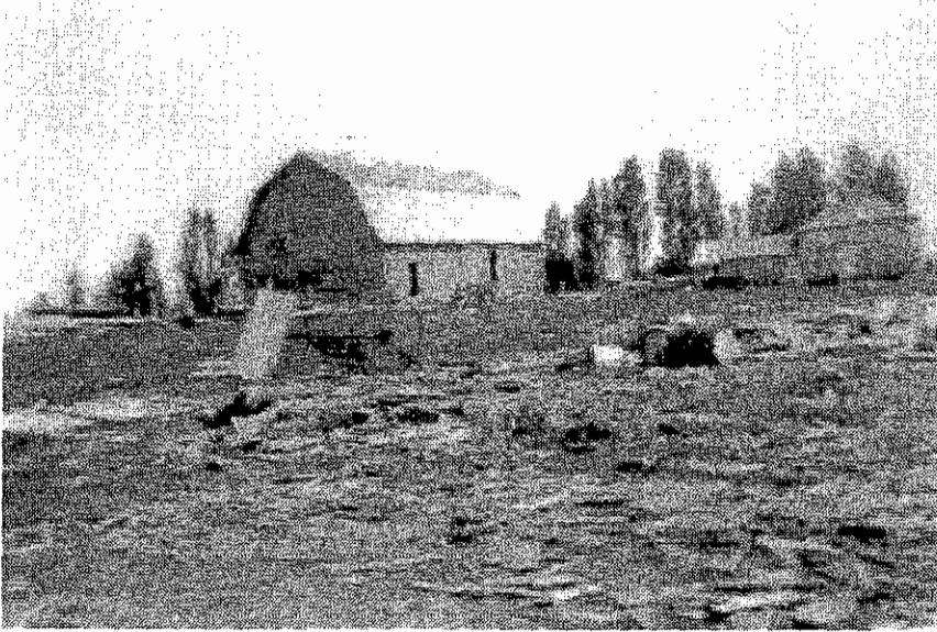
Figure 3.9. The partially-finished MIA barn at North Manitou Village, 1927. The completed barn housed the MIA dairy herd, farm equipment, hay, a cold storage room for deer carcasses, and ventilated lofts for temporary storage of cherries. The debris in the foreground may be from demolished buildings formerly utilized by the Boardmans and Newhalls.
