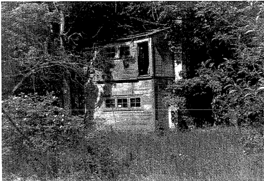
Figure 4.114. Margaret and Roderick Peattie treehouse, 1996. The two-story cottage built for Margaret and Roderick Peattie is one of the most curious structures on North Manitou Island. Unfortunately, the treehouse is deteriorating rapidly due to several decades of deferred maintenance.
