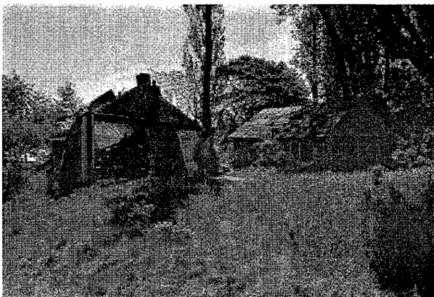
Figure 4.18. Manitou Island Association carpenter shop and machine shop, 1996. Like the large barn, the basement level of the carpenter and machine shops were integrated into the slope of the beach ridge. Although their cobblestone foundations remain intact, the wooden superstructures of both shops currently are in ruinous condition.
