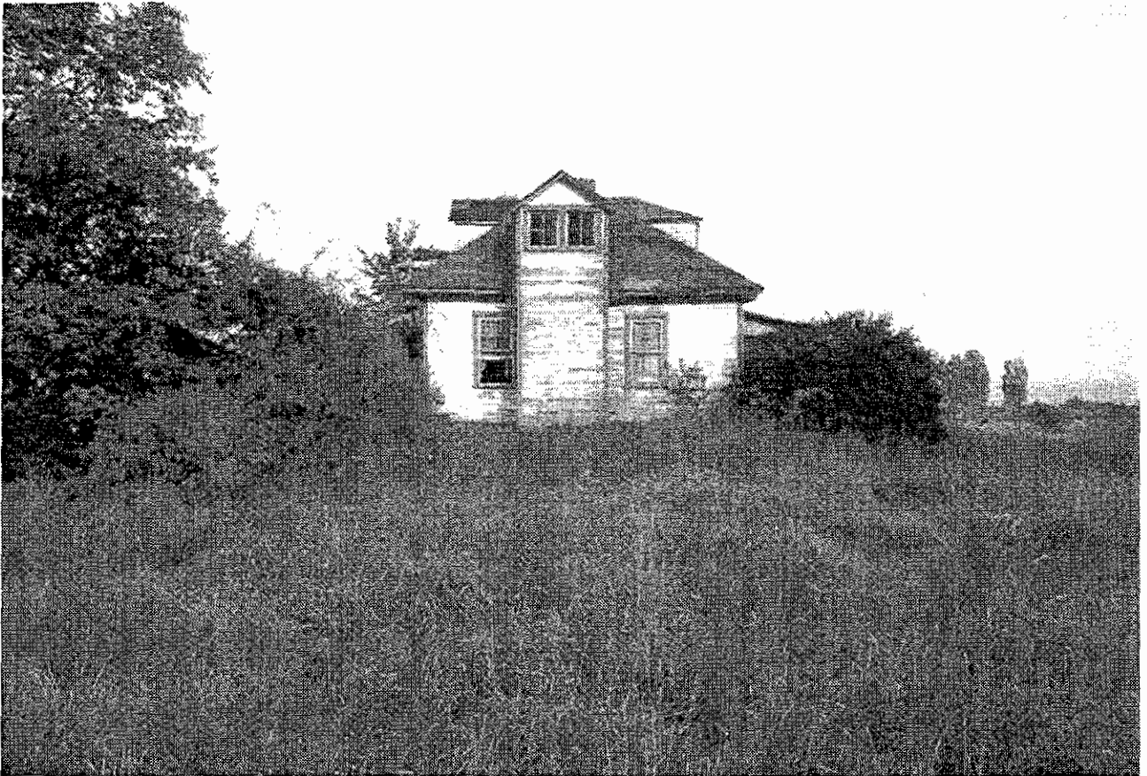
Figure 4.134. John Newhall cottage, western elevation, 1996.
