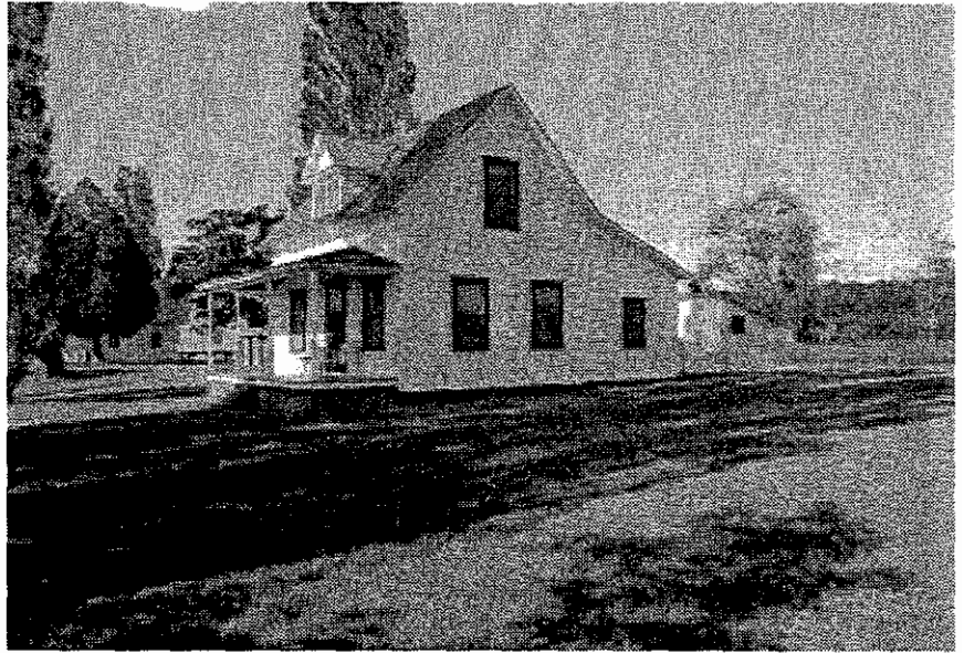
Figure 4.100. Hans Halseh House, U.S. Life Saving Service station, 1996. This simple, vernacular house is representative of the modest dwellings that USLSS crew members constructed for themselves and their families. Like other small structures at North Manitou Village, these houses tended to be highly mobile landscape features.
