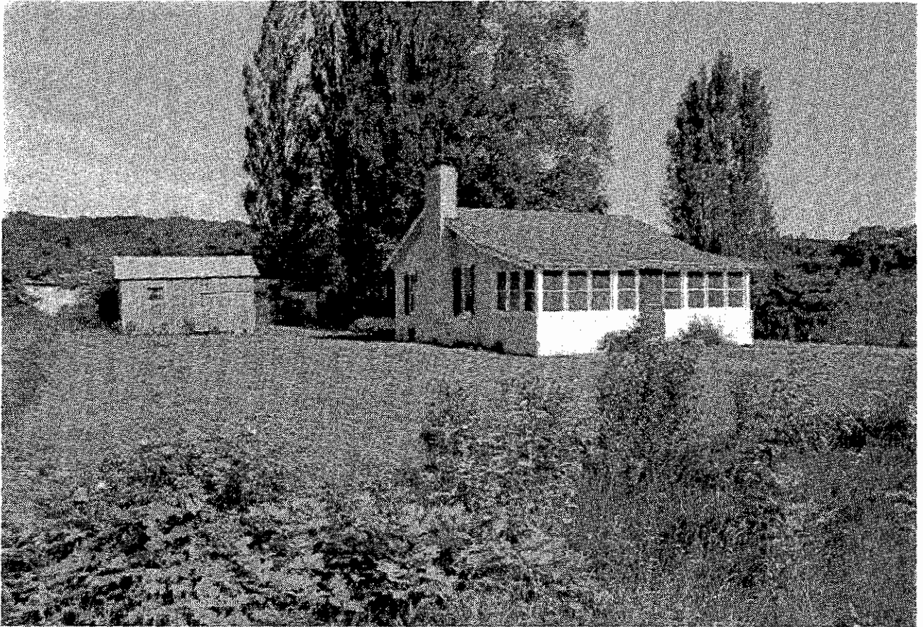
Figure 4.126. Shirley Foote Alford cottage and migrant orchard workers' cabin, 1996. A "mail-order" house, the Alford cottage represents a practical solution to the dilemma of constructing a building in a remote setting that, during the late 1930s, lacked both modern materials and a skilled labor force.
