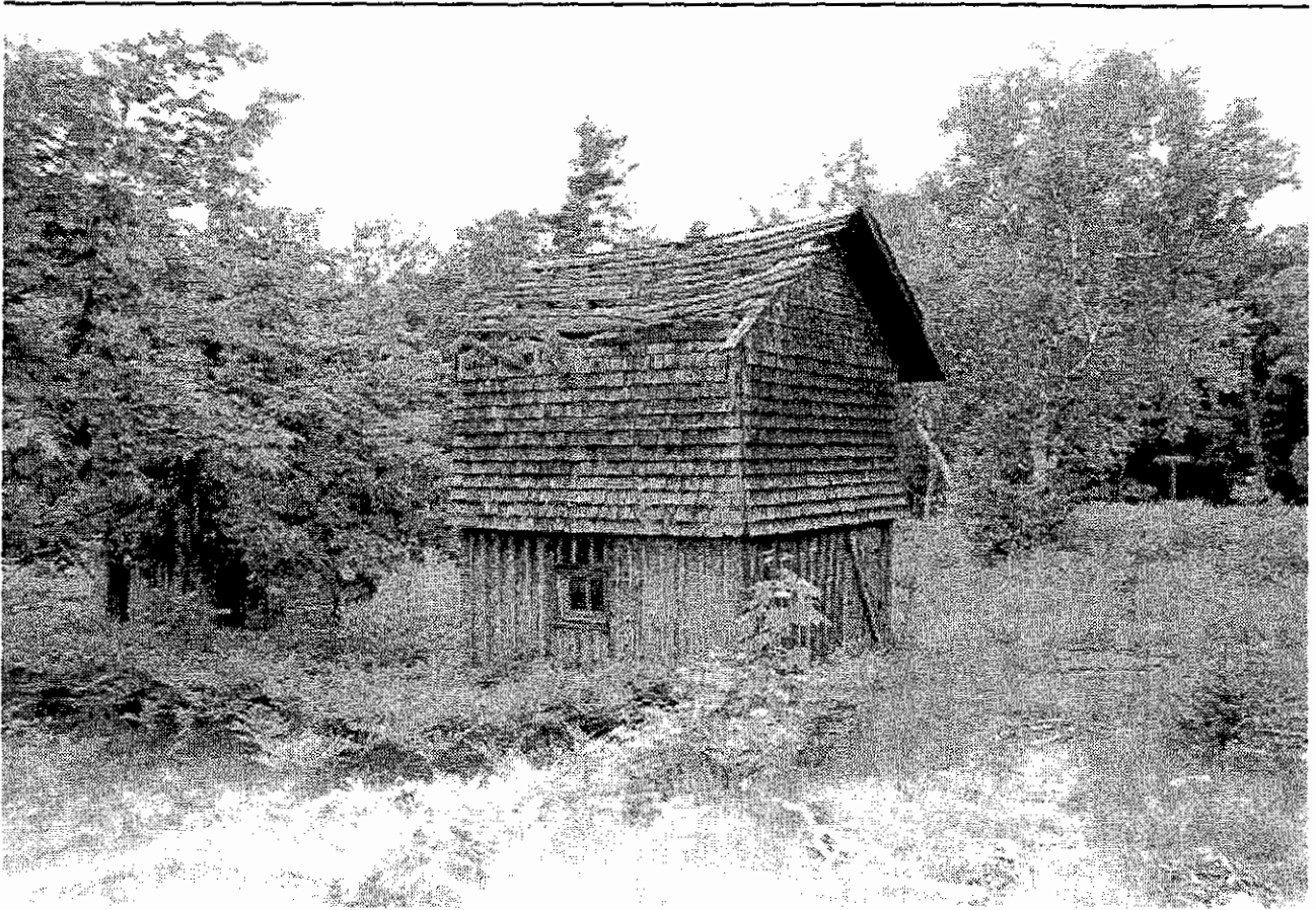
Figure 4.56. Alvar and Mary Bournique ice house, 1996. The Bournique ice house is one of the most visually intriguing structures on North Manitou Island. Its form, decoration, and exterior cladding materials complement the architecture of the residence.
