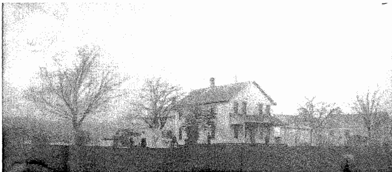
Figure 4.4. The “farmhouse,” ca. 1910s. This structure served as the Boardman family’s North Manitou home. The house subsequently was owned by the Newhall family, the Manitou Island Syndicate, and the Manitou Island Association. It was destroyed by fire sometime in the late 1920s.
