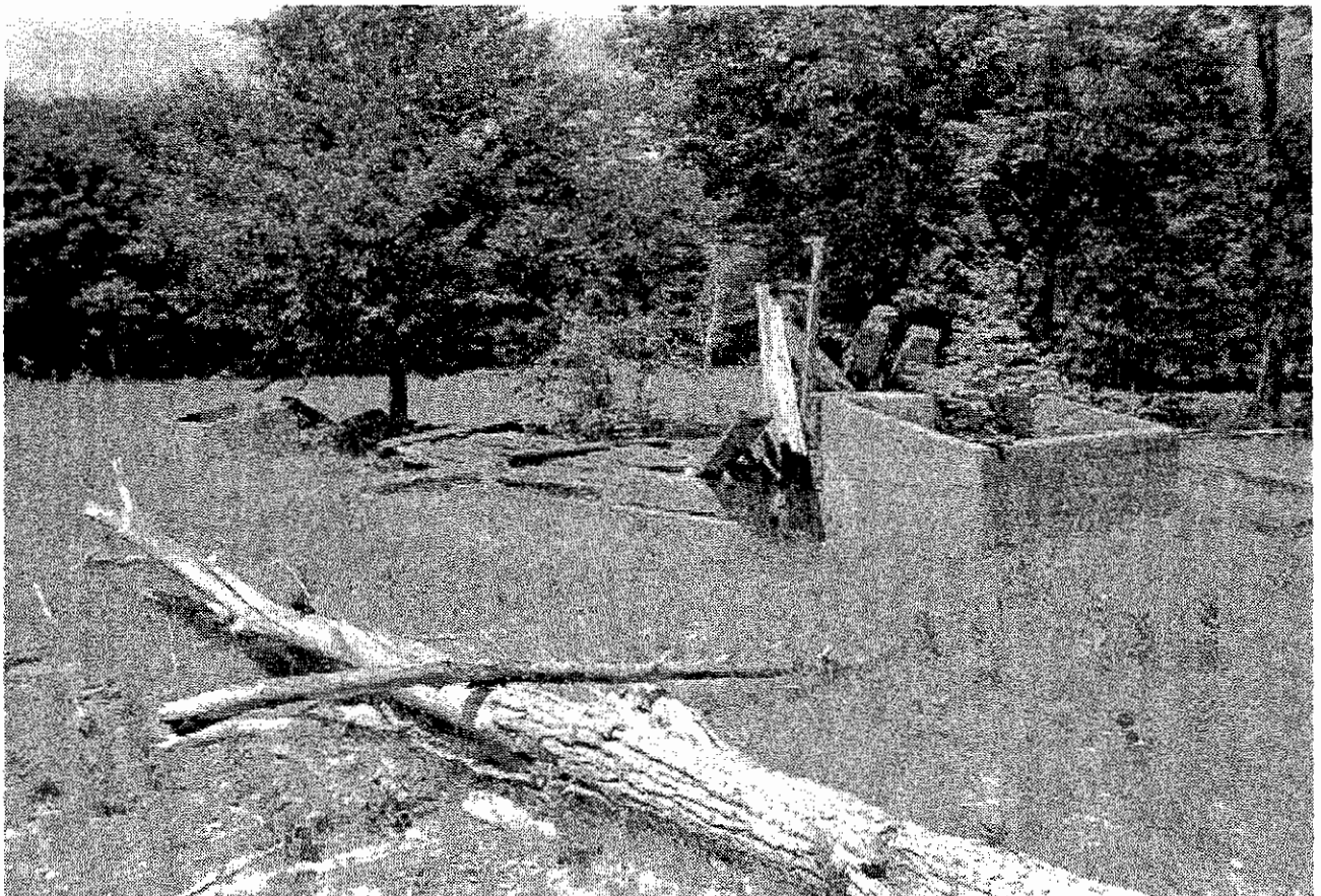
Figure 4.48. Concrete water troughs and foundation of large log barn, Alvar and Mary Bournique farm, 1996.
