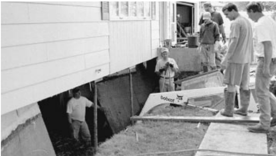
Workers braced a home in Garrison after June floodwaters buckled a basement wall.
