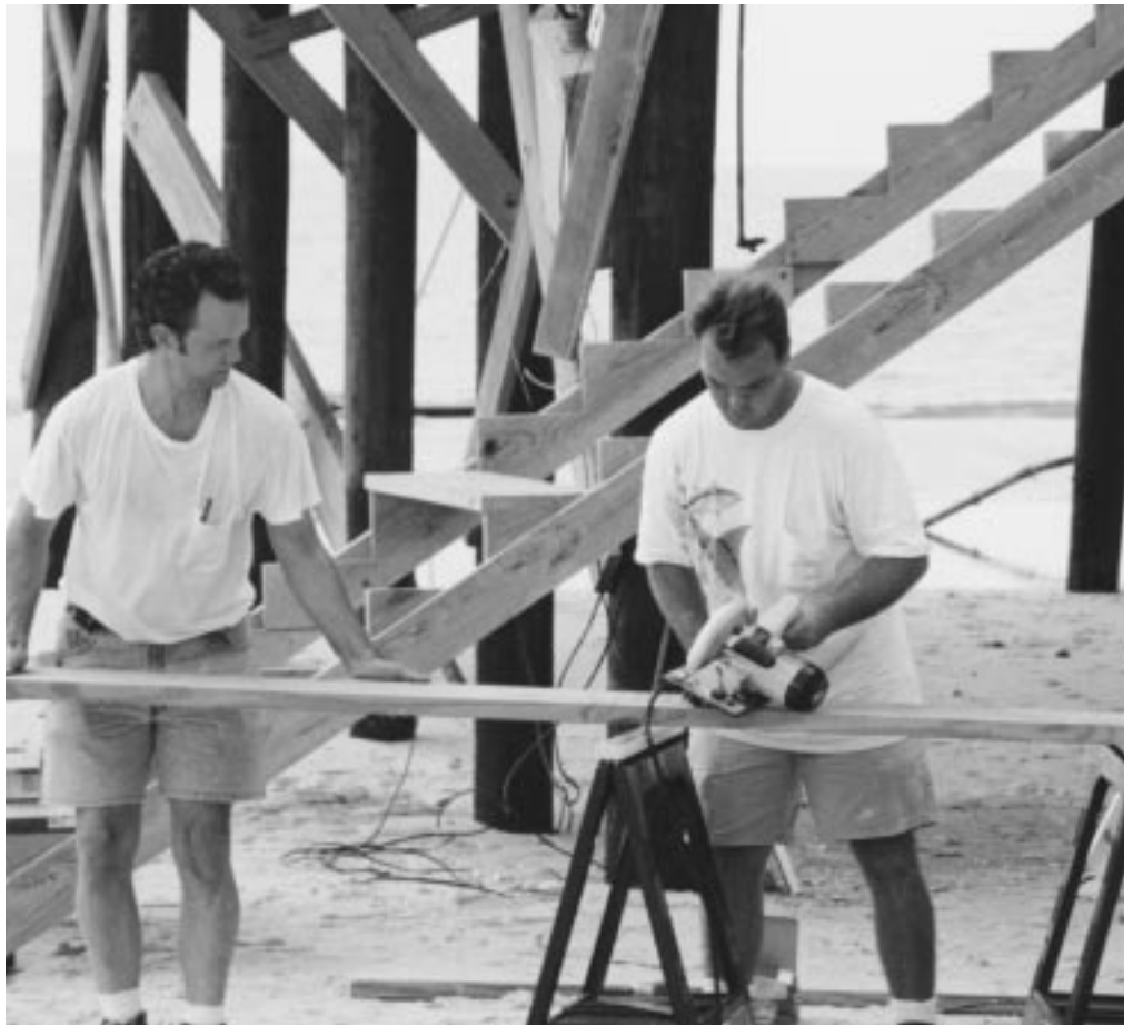
Repairs begin on damages from Hurricane Georges.
