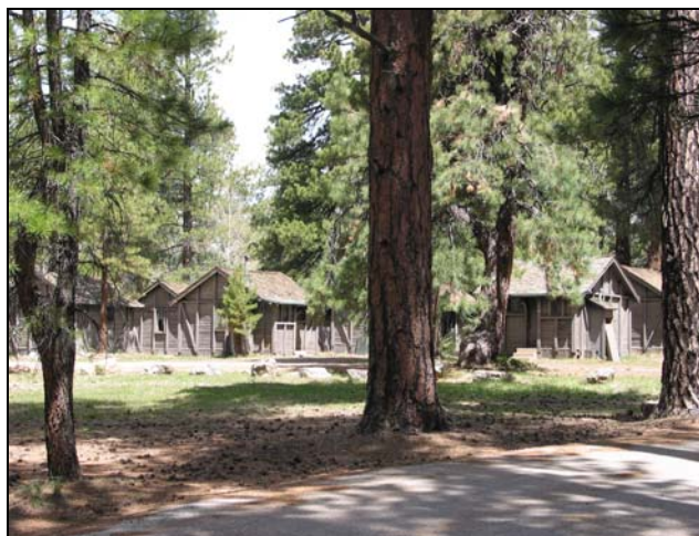
View of Exposed Frame Cabins
