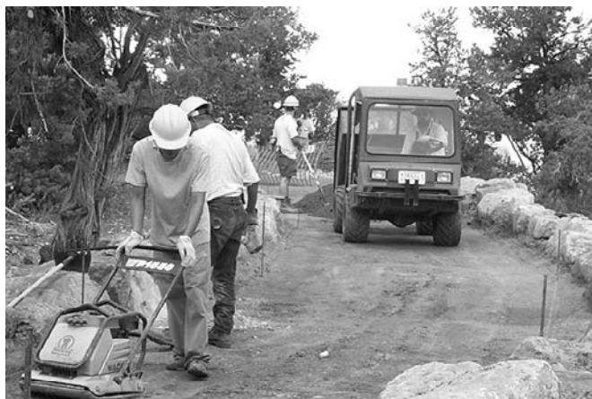
constructing the Greenway between Yavapai Observation Station and Mather Point
