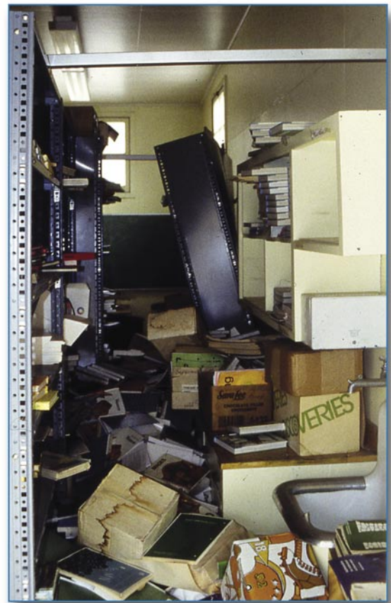
Figure 4-10 Fallen filing cabinets and shelves, Northridge, CA, 1994
