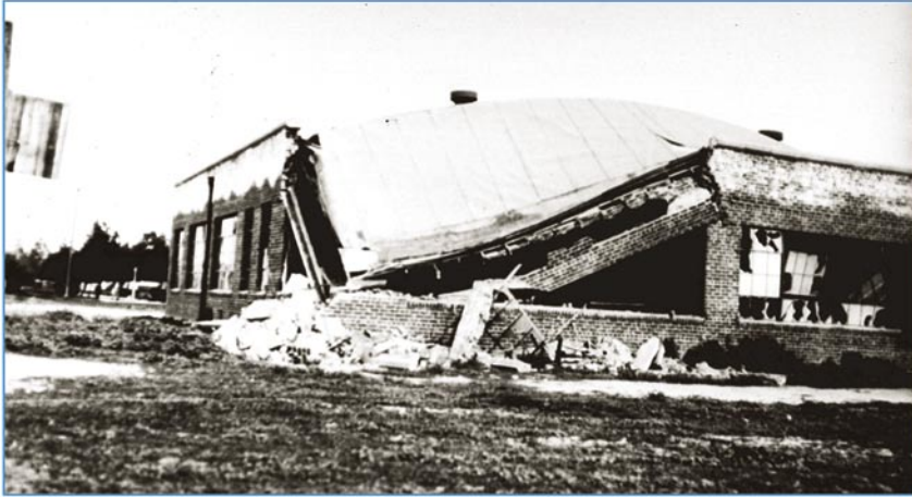
Figure 4-15 Damage to shop building, Compton Junior High School, Long Beach, CA, 1933
