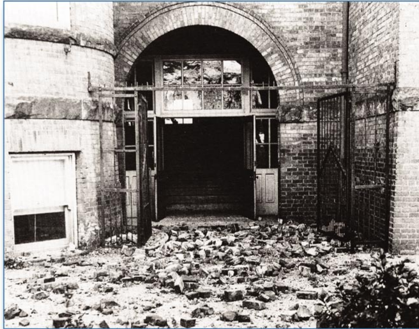
Figure 4-22 Another dangerous entry collapse, Seattle, WA, 1949
