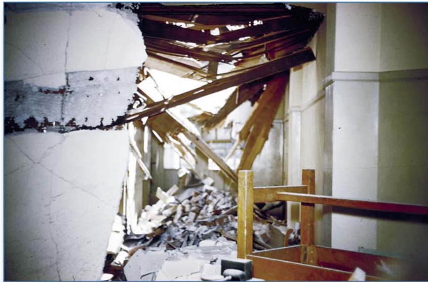
Figure 4-19 Destroyed exit corridor, Bakersfield, Kern County, CA, 1952
