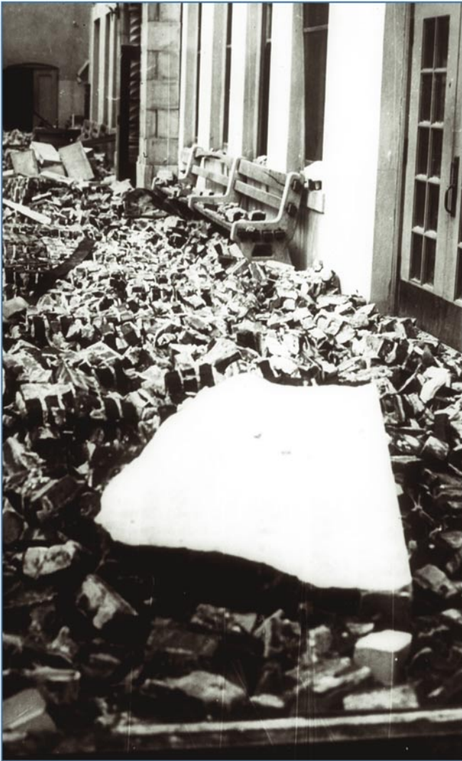
Figure 4-16 A dangerous passage way between two buildings, Polytechnic High School, Long Beach, CA, 1933
