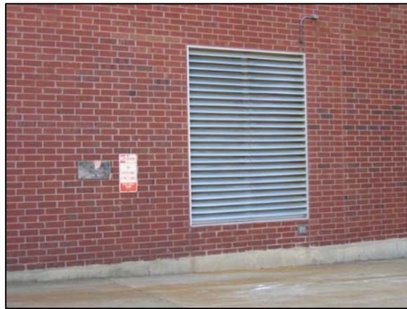
Figure 14. Air Intake
