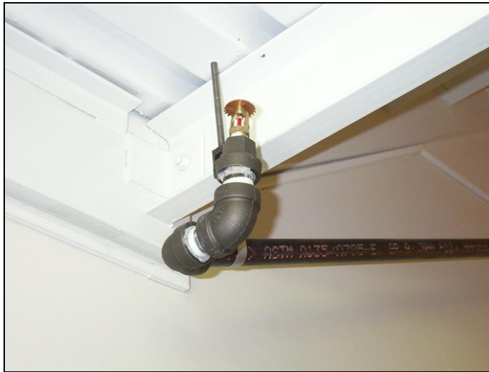
Figure 17. Sprinkler Head
