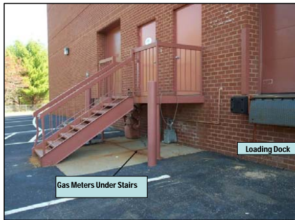
Figure 15. Loading Dock Area
