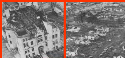
Tornado damage at the Monticello courthouse (left) and throughout the town of Monticello, IN (right).
