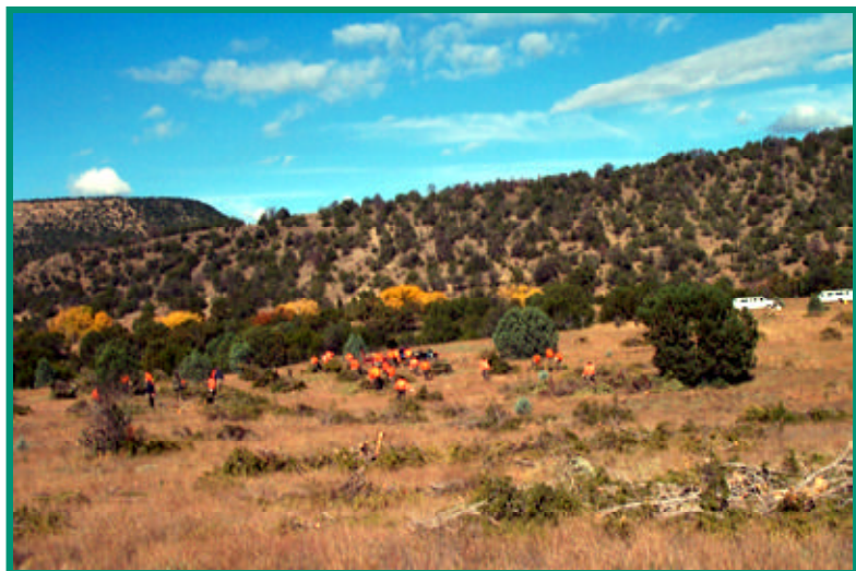
Youth Challenge squads build piles of debris for later burning.
