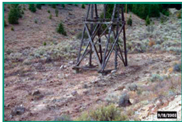
The same aerial tramway tower following fuels reduction treatment (one of ten treated).
