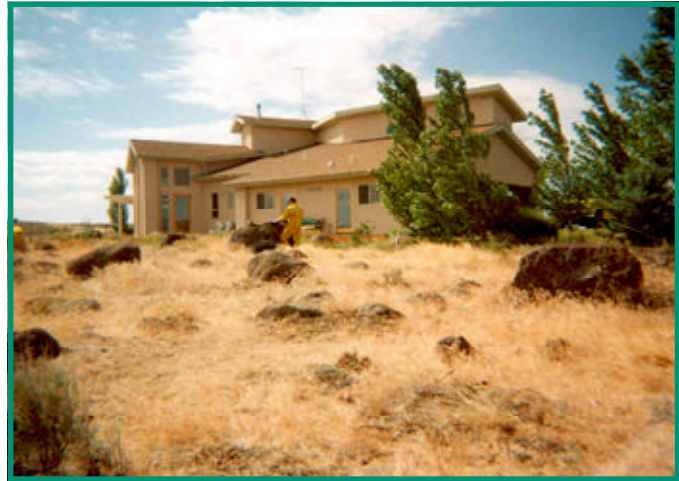
Banberry-Hidden Landing home following sagebrush removal. The small light fuels that remain will greatly reduce the intensity of any oncoming wildfire.
