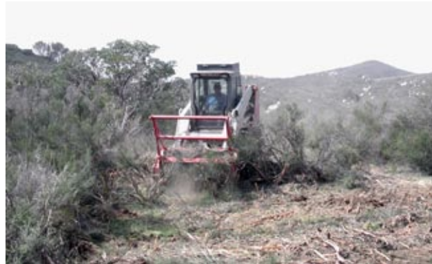
Mastication work at Poppet Flat.
