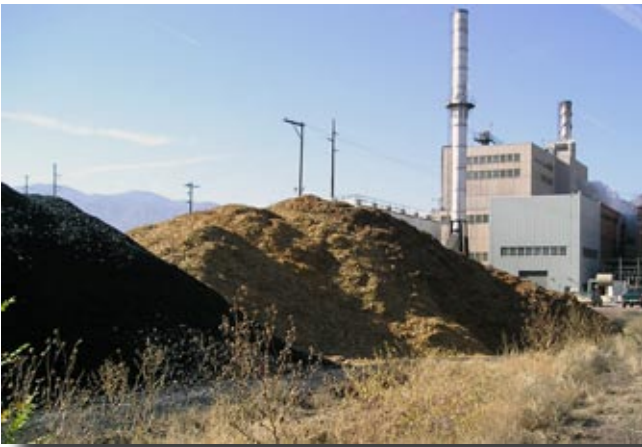
Biomass from BLM thinning project will be utilized by the Aquila Power Plant seen in the background.
