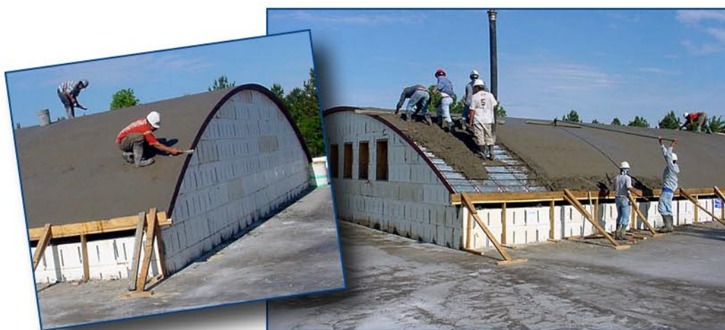
Construction of the steel-truss roof system.
