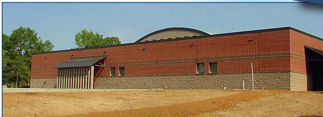
Completed reinforced ICF walls.
