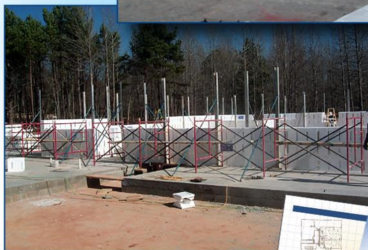
Erection of the reinforced ICF walls.
