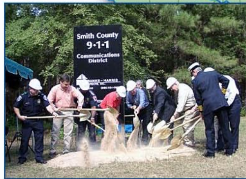
Ground clearing and construction of the Smith County 911 Communications Dispatch and Emergency Operations Center began in mid-October 2002.
