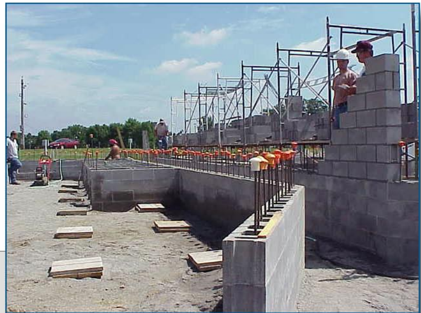
Construction of reinforced CMU interior partition fully reinforced CMU walls.
