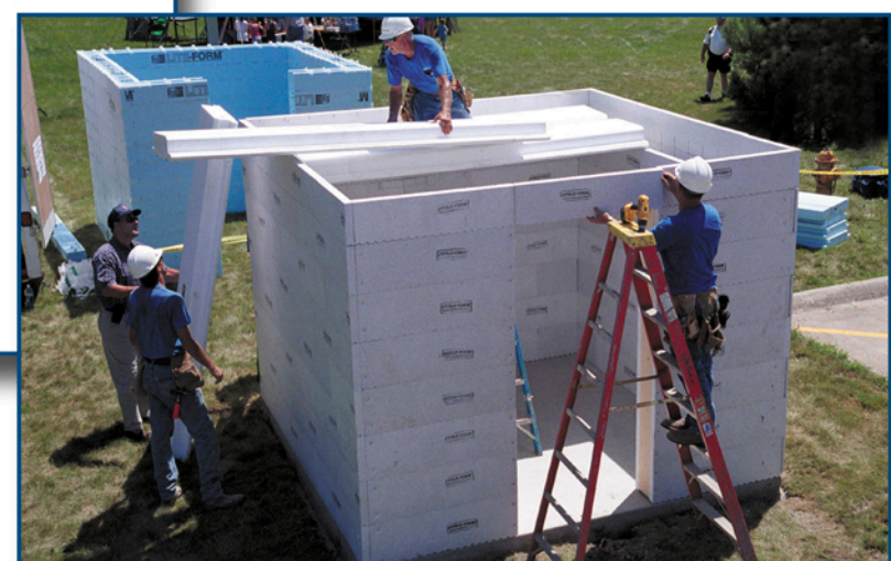
Workers assemble the roof panels, which will be covered with rebar and concrete.
