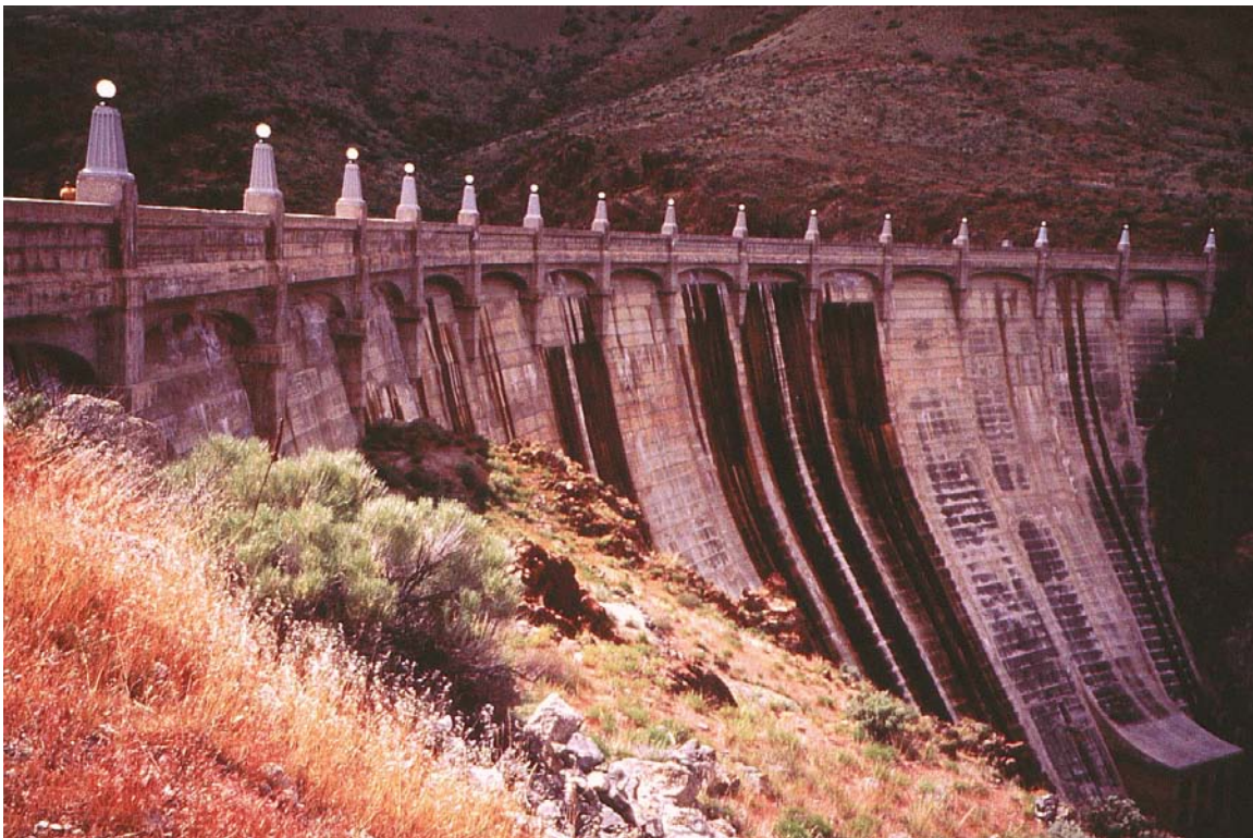
Figure 1a.—Owyhee dam seen from the right abutment.
