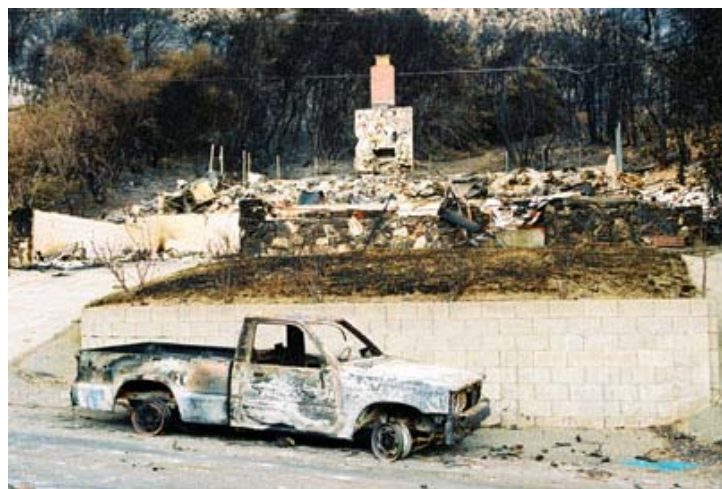
A burned pickup truck and stone foundation are all that remain of a home in Waterman Canyon. (DHS-FEMA)
