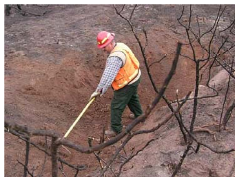
A BAER Team member clearing a culvert (U.S. Park Service)
