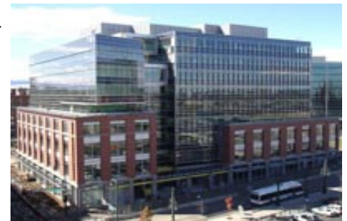
EPA Region 8’s facility in Denver includes many design features and systems that dramatically reduce energy use and greenhouse gas emissions.
