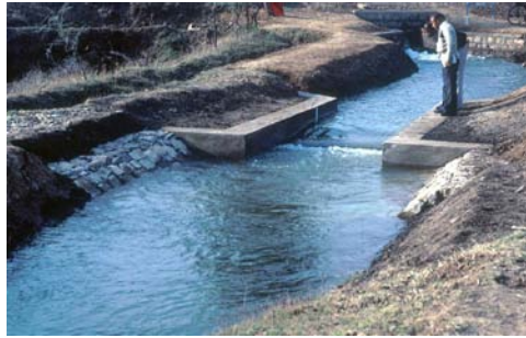
Figure 5. — A Rectangular-Throated Flume in India.
