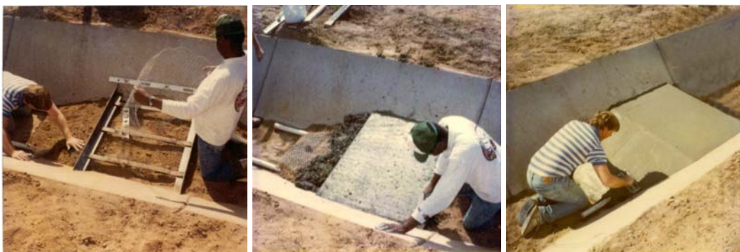
Figure 2. — Construction of a Broad-Crested Weir in a Concrete-Lined Trapezoidal Channel.
