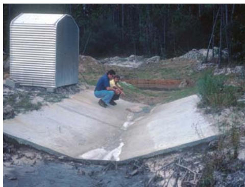
Figure 6. — Triangular-Throated Flume in Florida.
