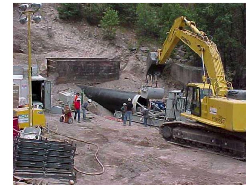
The U.S. Army Corps of Engineers installed a new 84-inch diameter culvert through the Diamond Ave. fill bridge to reduce risk of breach and protect municipal infrastructure
