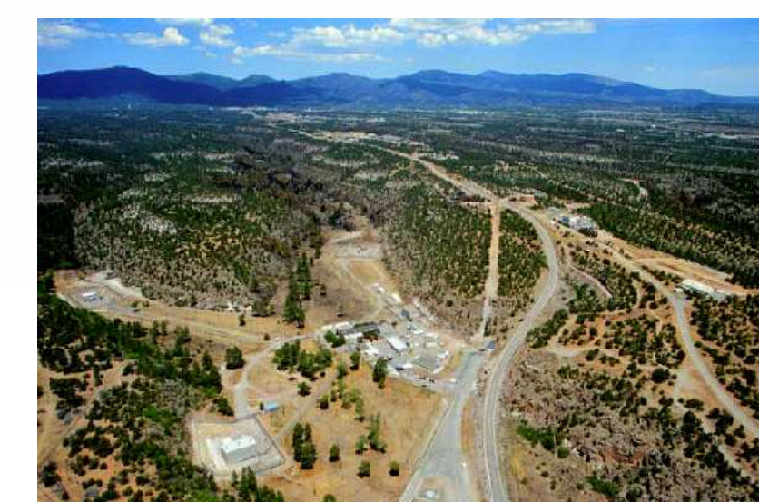
Nuclear research facilities in Pajarito Canyon are now protected by the flood-control dam
