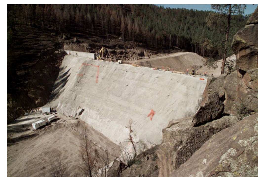
New RCC flood and debris-control dam constructed by U.S. Army Corps of Engineers in Pajarito Canyon
