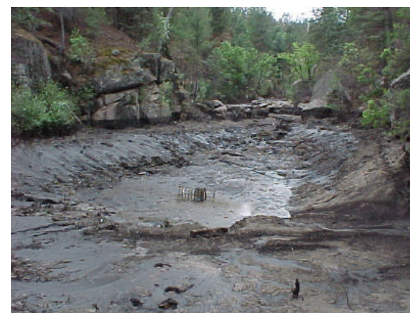
Upstream side of Diamond Ave. roadfill – existing 18-inch culvert after June 2, 2000 storm
