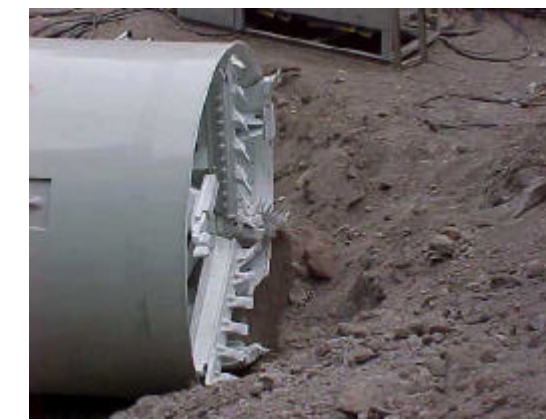
The U.S. Army Corps of Engineers installed a new 84-inch diameter culvert through the Diamond Ave. fill bridge to reduce risk of breach and protect municipal infrastructure
