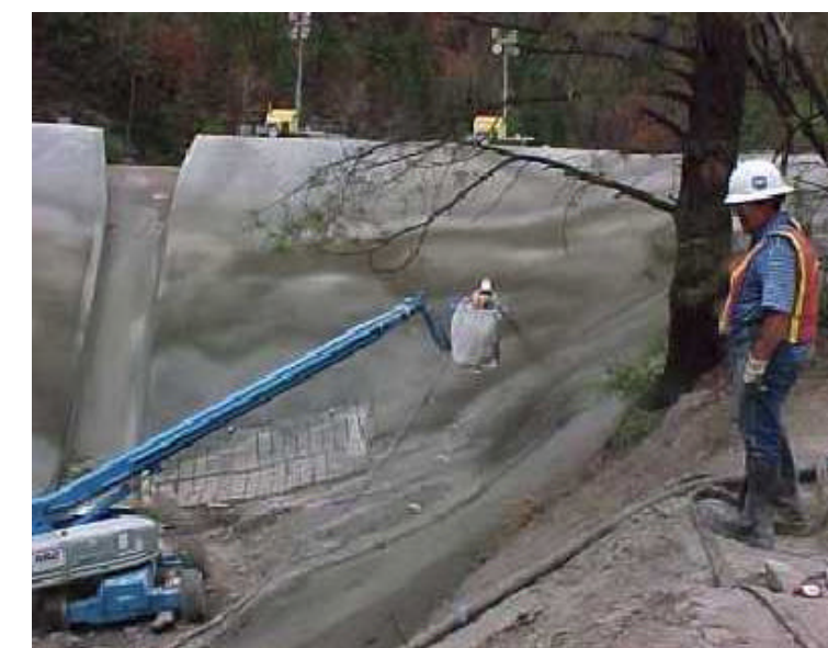
Applying shotcrete protection to Los Alamos Dam
