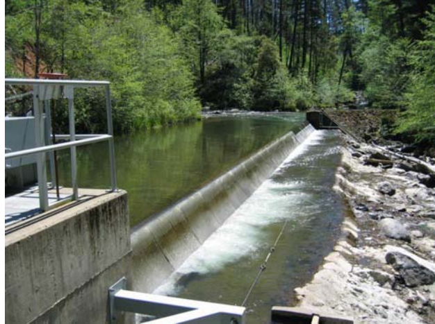
Figure 9. — Montgomery Creek intake.
