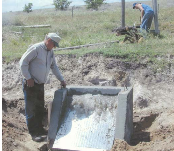
Figure 5. — Coanda-effect screen structure similar to that shown in Fig. 4, operating at a relatively high flow rate. All flow still passes through the screen before reaching the toe.
