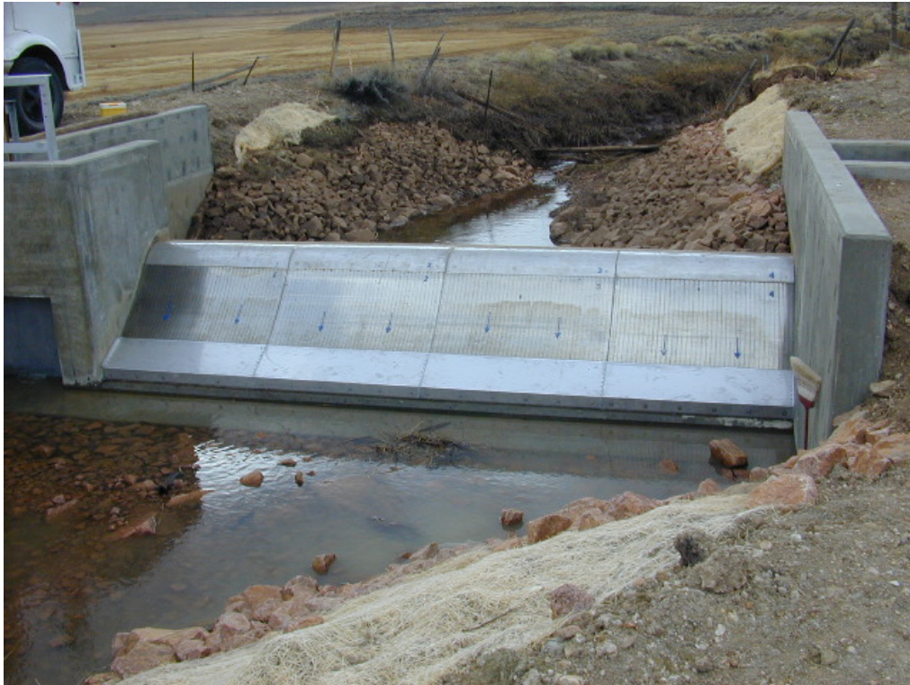
Figure 7. — Coanda-effect screen structure at Lake John, constructed in 2001. This structure replaced that shown in Fig. 6.
