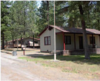
Fire stations are only a part of the infrastructure on the Modoc National Forest — Other structures include lookouts, office buildings, refrigerated tree coolers and storage buildings
