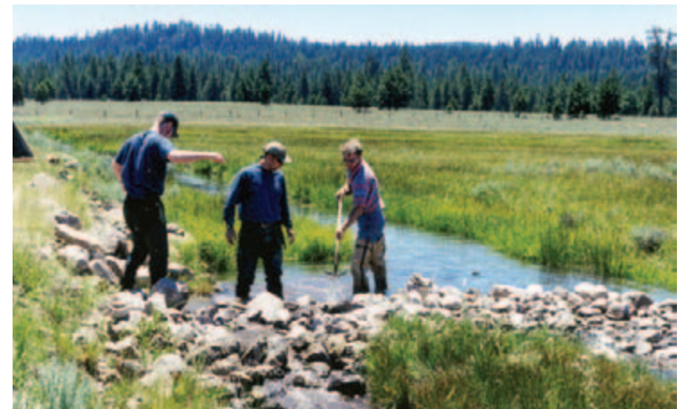
Creating a diversion of water into historic channel on Pine Creek
