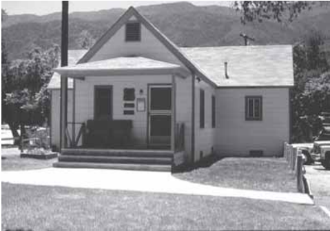
Built around 1935, this Series E Civilian Conservation Corps (CCC) administrative building is located at Oak Grove on the Palomar Ranger District.
