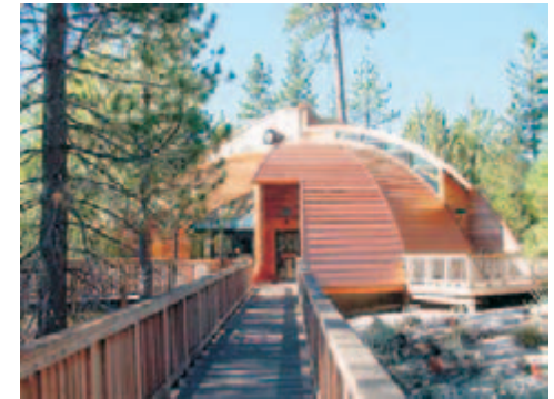
Chilao Visitor Center along the Angeles Crest Highway.
