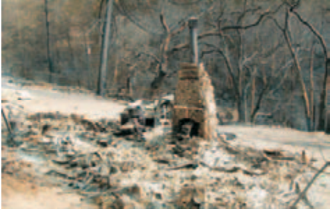
An historic cabin burned during the Williams Fire in 2002. Severe wildfires have destroyed many structures over the past several years.
