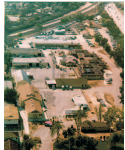
Aerial view of the ANF Supervisor's Office.
