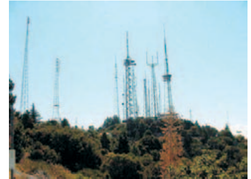
Telecommunications towers on an ANF mountaintop are operated under special use permits.
