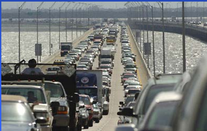
Howard Franklin Bridge, Pinellas County Florida
