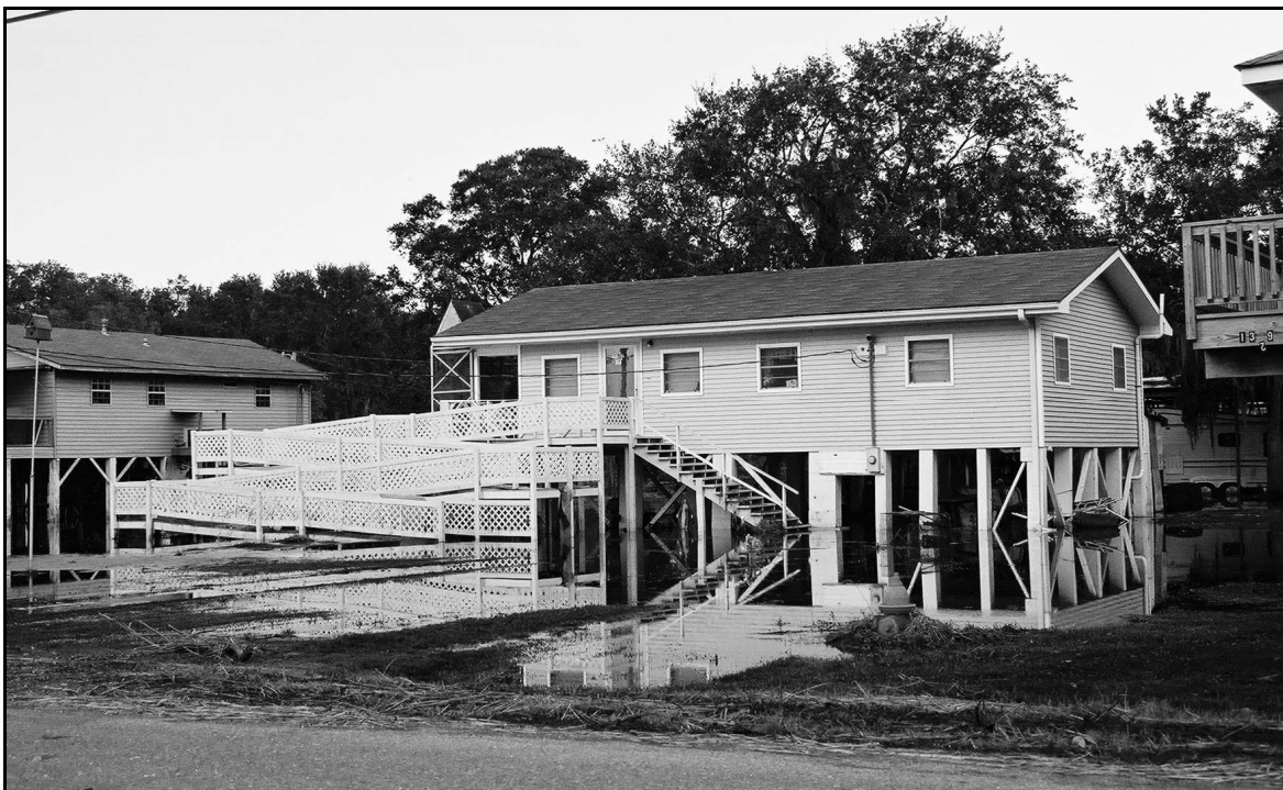
Figure 5. Accurate flood hazard maps are essential for the application of appropriate construction standards, such as elevation above the flood level.
