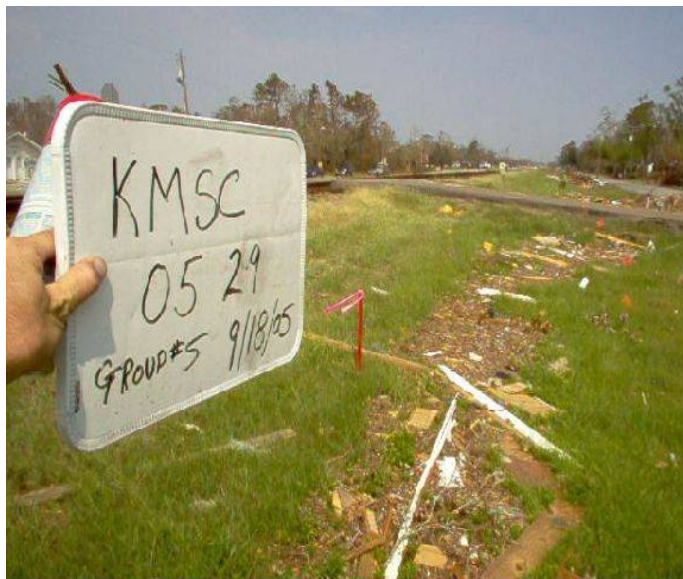
Figure 8 – Debris Line HWM
