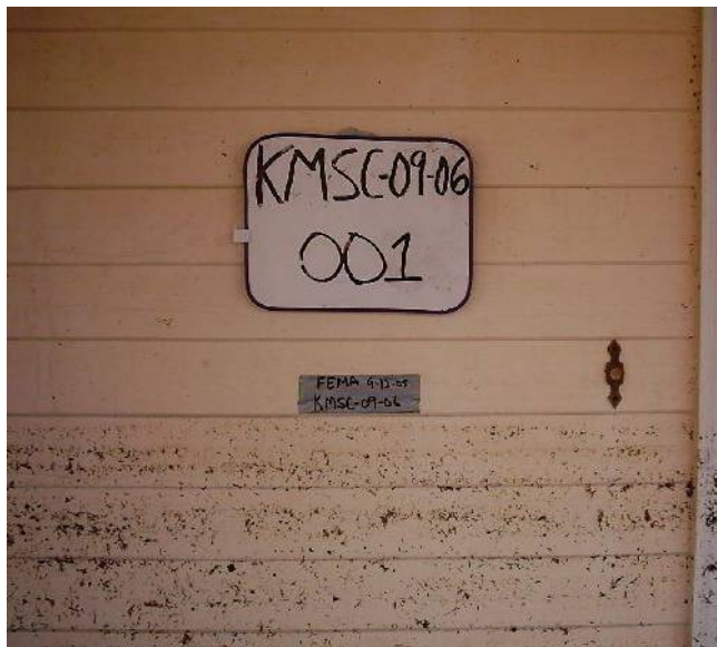
Figure 7 – Exterior Mud Line HWM
