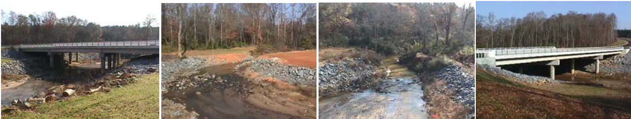
Figure 6. Examples of Bridge Photographs
