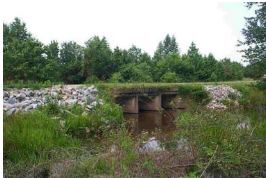
Figure 48. Example of Approximate Survey Photograph
