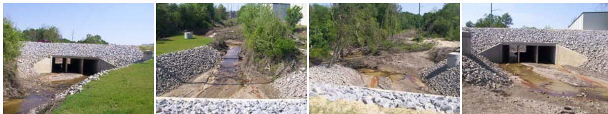
Figure 18. Examples of Culvert Photographs
