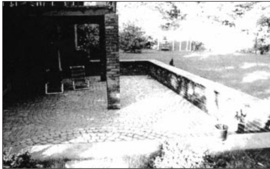
Figure 3-12 House protected by a floodwall designed as a landscaping feature.
