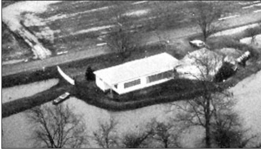
Figure 3-11 House protected by levee, which holds back the flood waters shown in the lower half of the photograph. Note that the levee ties in to high ground created by the road embankment.
