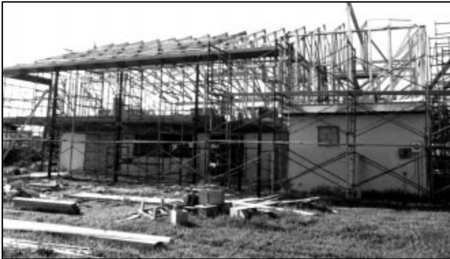
Figure 3-6 The owner of this floodprone house in south Florida decided to build a new frame second story on top of his masonry first story. The new second story is well above the BFE.
