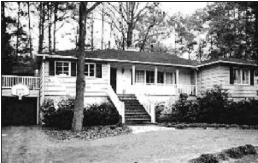
Figure 3-4 Retrofitted house elevated on extended continuous foundation walls.
