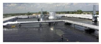
An emergency roof (shown) was installed after Hurricane Charley blew the mechanically attached PVC membrane roof covering off the concrete deck of the Fawcett Memorial Hospital.
