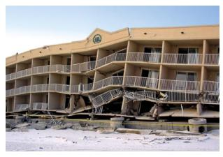
A multi-family condominium collapsed after Hurricane Ivan due to erosion of supporting soil under the shallow foundation.
