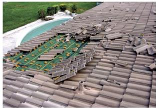
In addition to the damage shown in this photo, this one-story roof lost virtually all of the hip and ridge tiles during Hurricane Charley. (Punta Gorda Isles)
