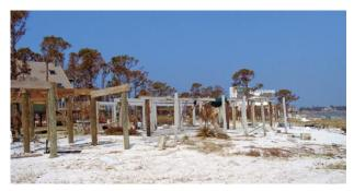
Several structures were completely torn off their pile foundations during Hurricane Ivan as a result of significant flood depths, waterborne debris impacts, and lack of connections.
