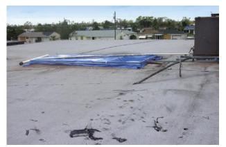
A large HVAC package unit was blown off this curb during Hurricane Charley. Note the loose LPS conductors this side of the curb. This school had significant damage from several pieces of rooftop equipment that blew off the building roof. (Port Charlotte Middle School)
