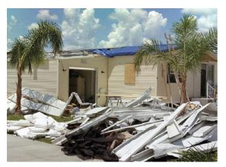
Manufactured housing that had structural damage resulting from accessory structure failure.
