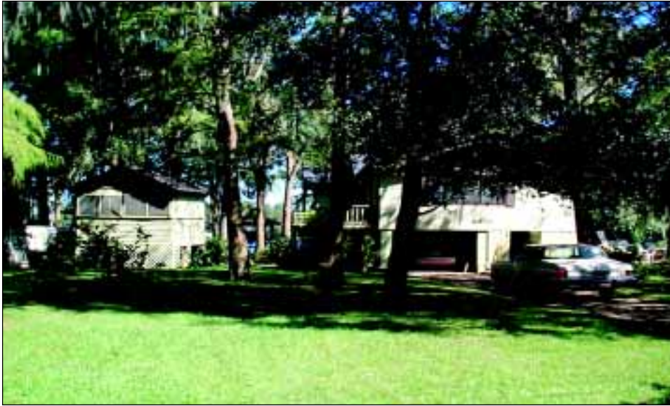
FIGURE 4-4 Elevated house along the Dog River that suffered minimal flood damage.
