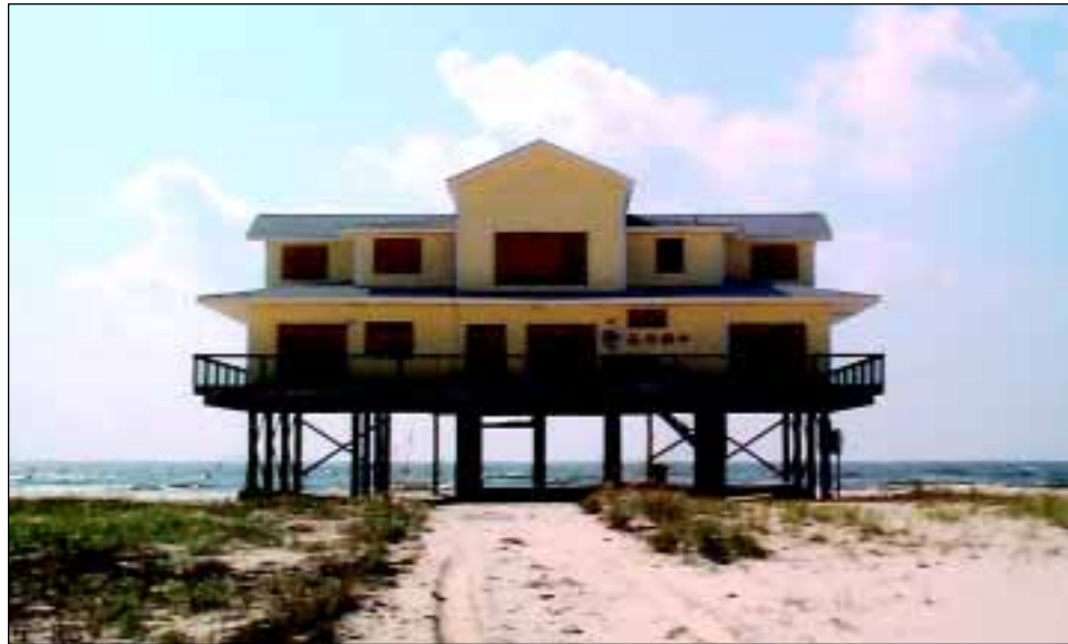
FIGURE 4-18 This house sustained no damage with the exception of loss of stairs and items stored below the first-floor elevation.
