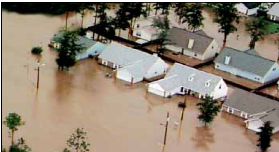
FIGURE 3-1 Houses inundated by 2 to 3 feet of floodwaters in the Florida Panhandle.
