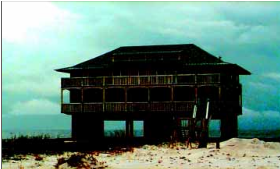
FIGURE 4-27 This properly elevated structure in Gulf Shores suffered no damage other than the loss of breakaway walls and slight damage to its stairs.
