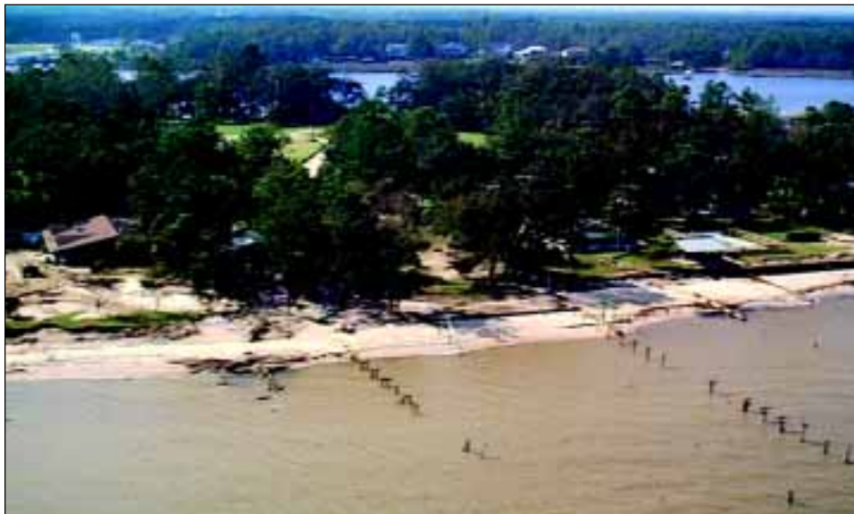
FIGURE 4-28 Typical shoreline erosion along low-lying areas adjacent to Mobile Bay.
