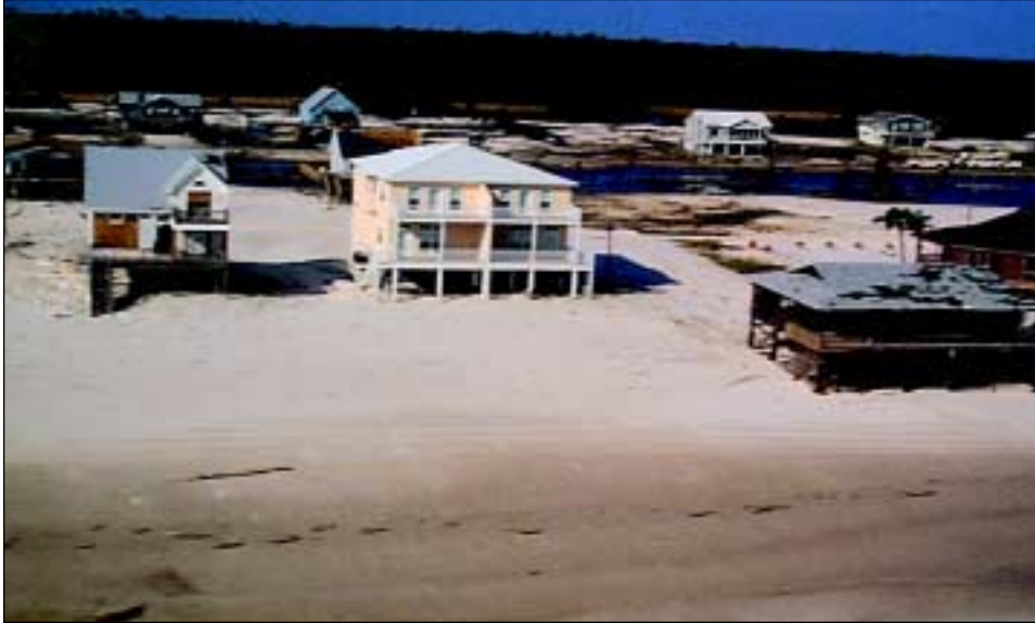
FIGURE 5-9 The structures to the left were elevated and set back and performed well.
