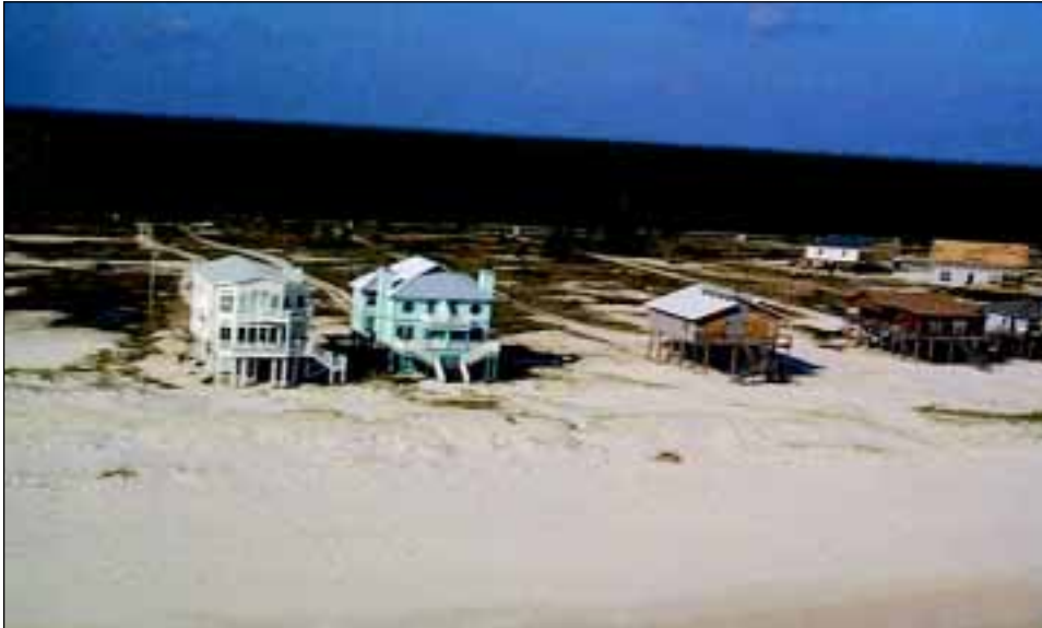
FIGURE 3-10 Properly elevated and set back houses sustained little damage.
