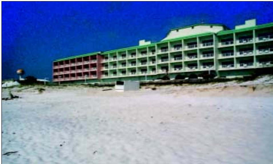
FIGURE 5-12 A newer hotel with an elevated first floor that suffered minimal damage.
