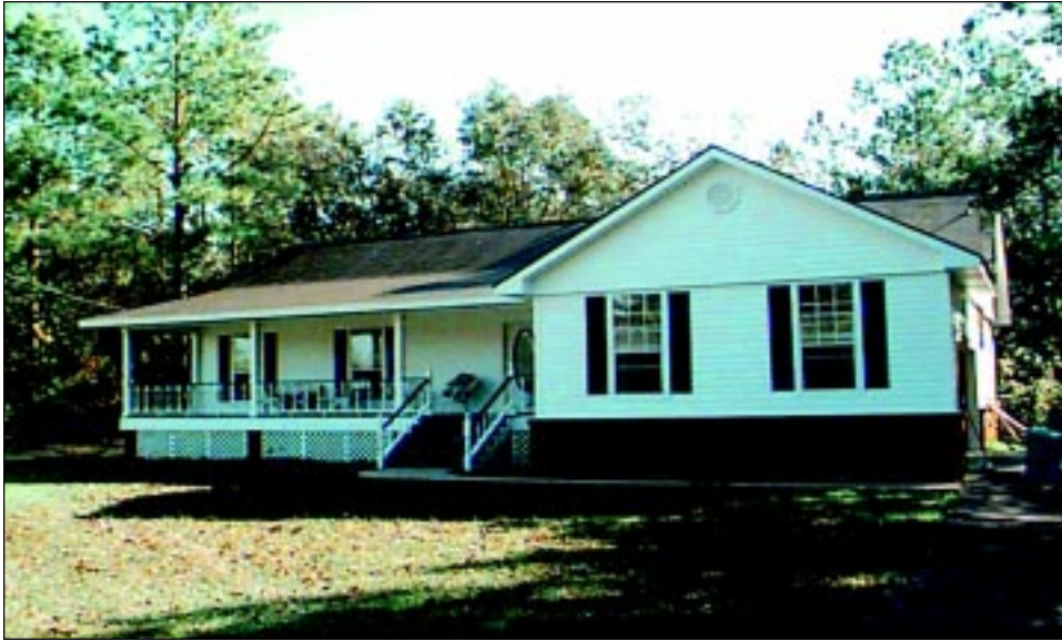
FIGURE 6-4 Home in eastern Jackson County elevated approximately 40 inches.
