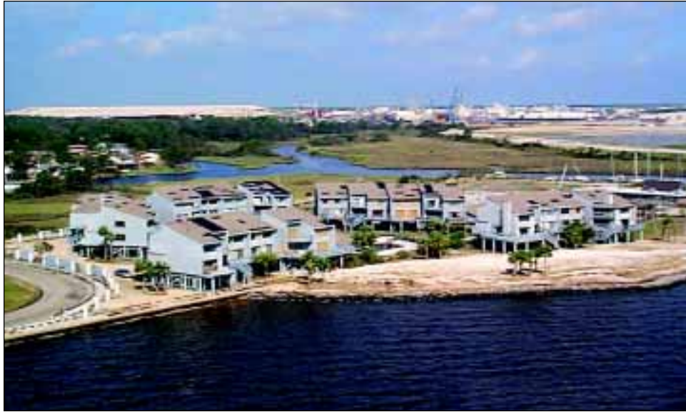
FIGURE 3-11 These condominiums near Pascagoula, Mississippi suffered wind damage to roofing shingles and siding.
