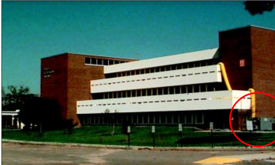
FIGURE 6-19 Mississippi Gulf Coast Community College in Gautier, where restoration services are underway to dry out interior areas.
