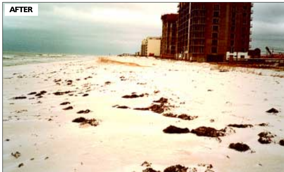
FIGURE 5-8 Navarre Beach after Hurricane Georges. Note the loss of revegetated dune.
