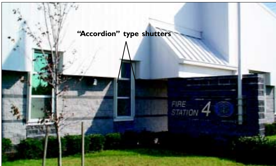
FIGURE 5-14 Window shutters on the Pensacola Fire Station No. 4.
