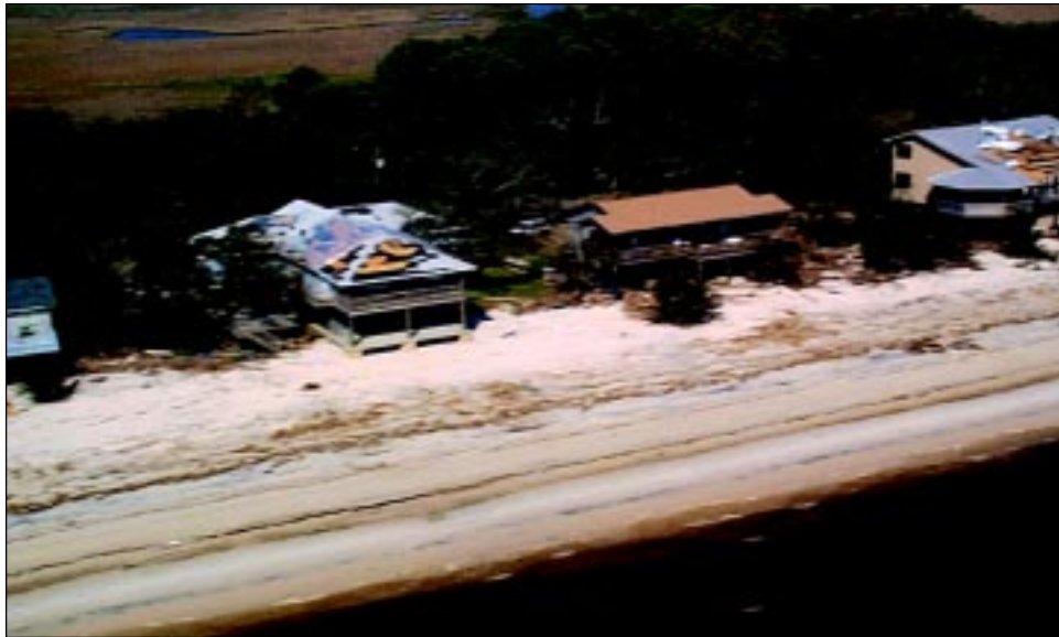
FIGURE 6-21 Shingle roof damage to homes along the open Mississippi coast.
