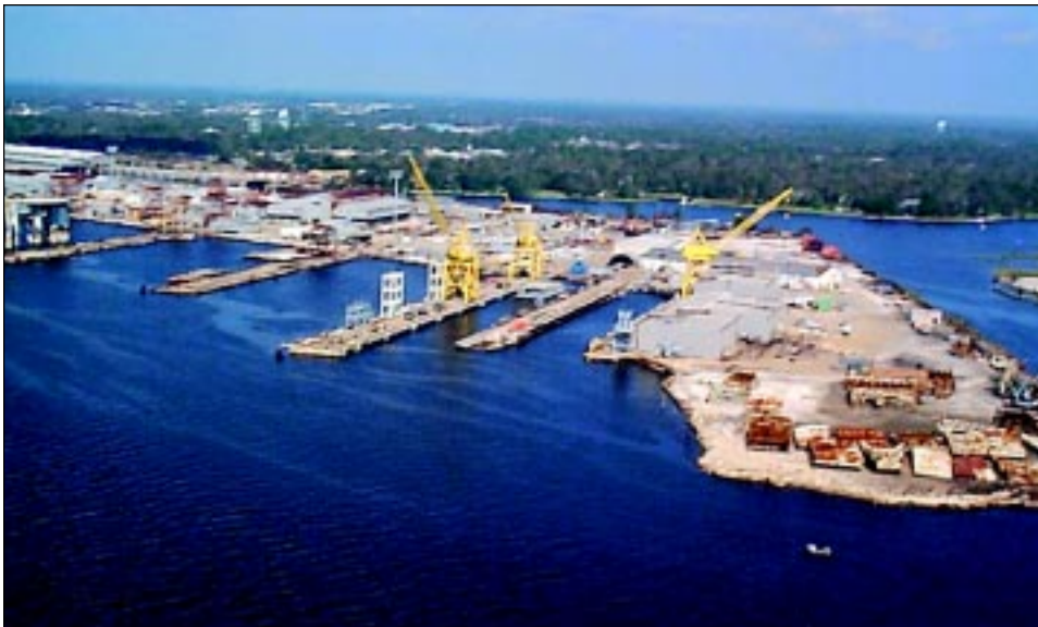
FIGURE 6-9 Ingalls shipyard only suffered minor damage due to coastal storm surge.
