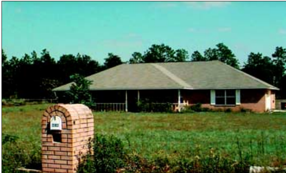
FIGURE 5-1 Repetitively flooded home slated for acquisition under FEMA’s HMGP.
