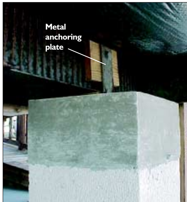
FIGURE 5-19 Reinforced masonry pier with metal anchoring plate.
