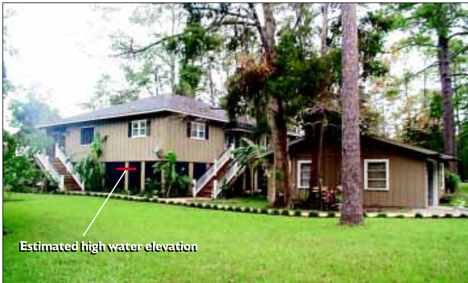
FIGURE 4-5 House along the Fish River, elevated through FEMA's HMGP that suffered minimal flood damage.
