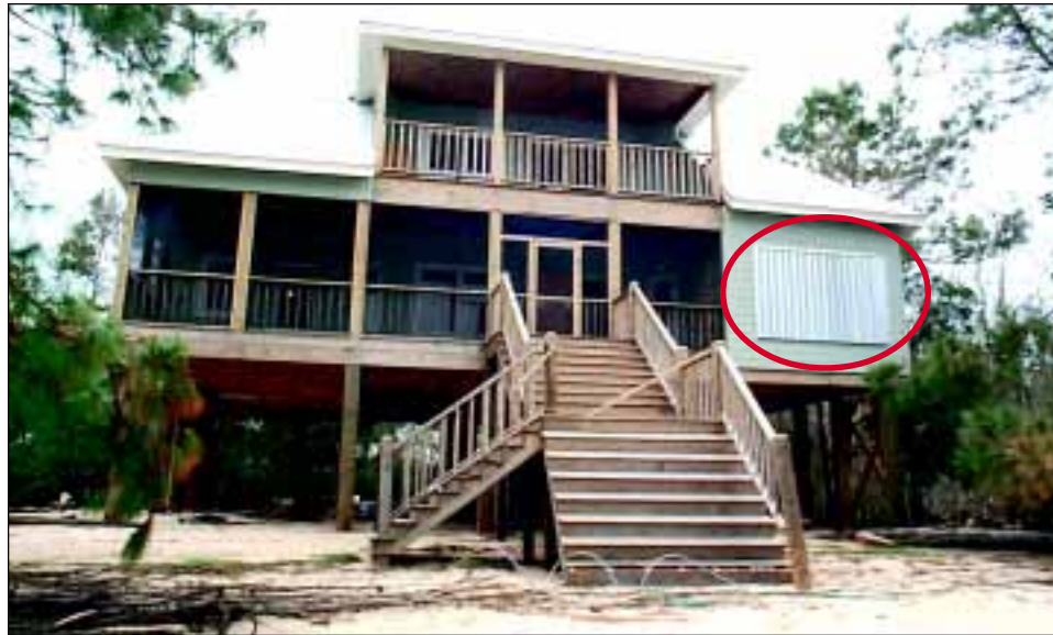
FIGURE 4-33 A properly elevated post-FIRM front-row coastal house that suffered only minor damage to stairs. Note the storm shutter on the front window.
