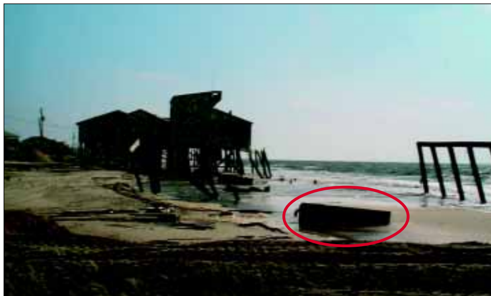
FIGURE 4-19 Old concrete septic tanks (circled) and drain fields have been superseded by the new municipal sanitary sewer system. The old systems still create a hazard as waterborne debris.
