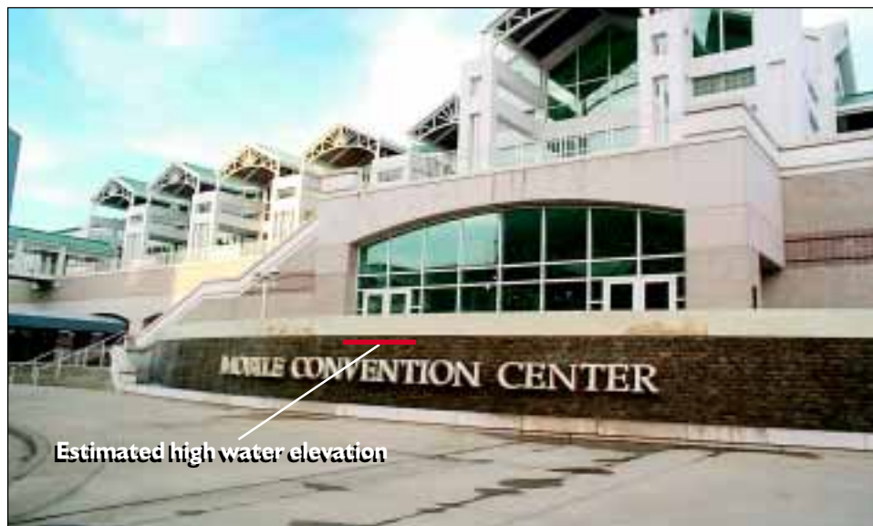
FIGURE 4-7 Despite approximately 7 feet of flooding in this area, the Mobile Convention Center suffered only minor damage and was operational when the floodwaters receded.
