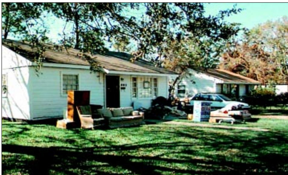
FIGURE 6-2 Typical pre-FIRM at-grade house flooded several feet in Pascagoula.
