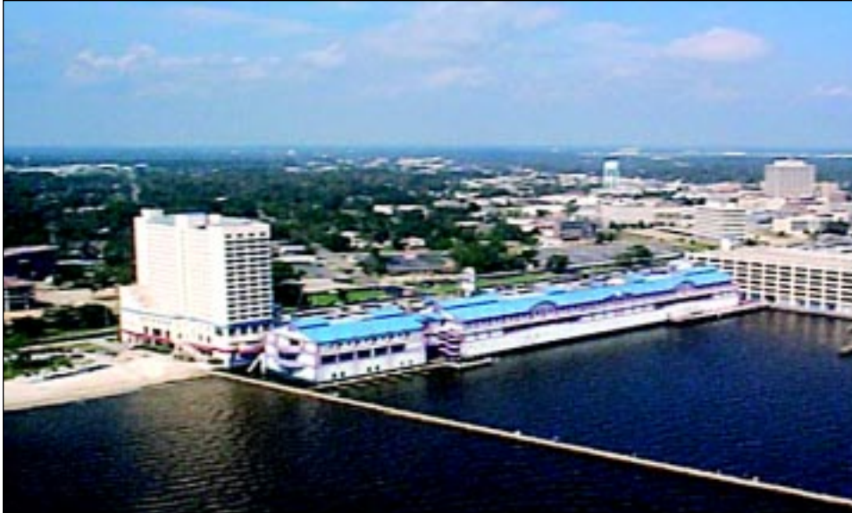
FIGURE 6-8 Casinos suffered minimal damage from coastal storm surge.
