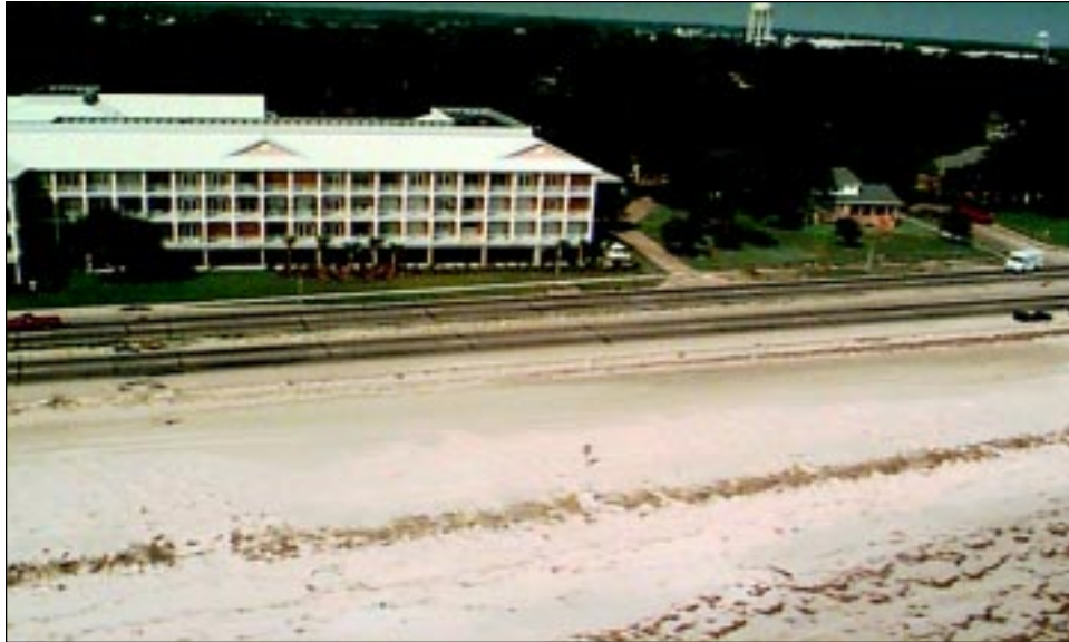
FIGURE 6-6 Coastal area near Gulfport. Note how buildings are set back from the shore.
