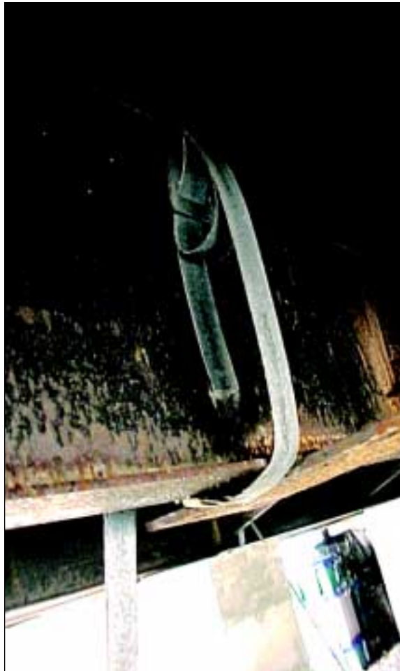
FIGURE 5-25 Proper strap installation.
