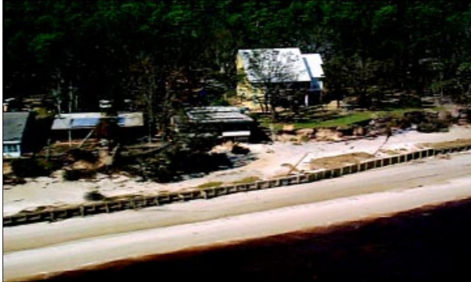
FIGURE 6-11 Severe beach erosion caused by wave action and storm surge.
