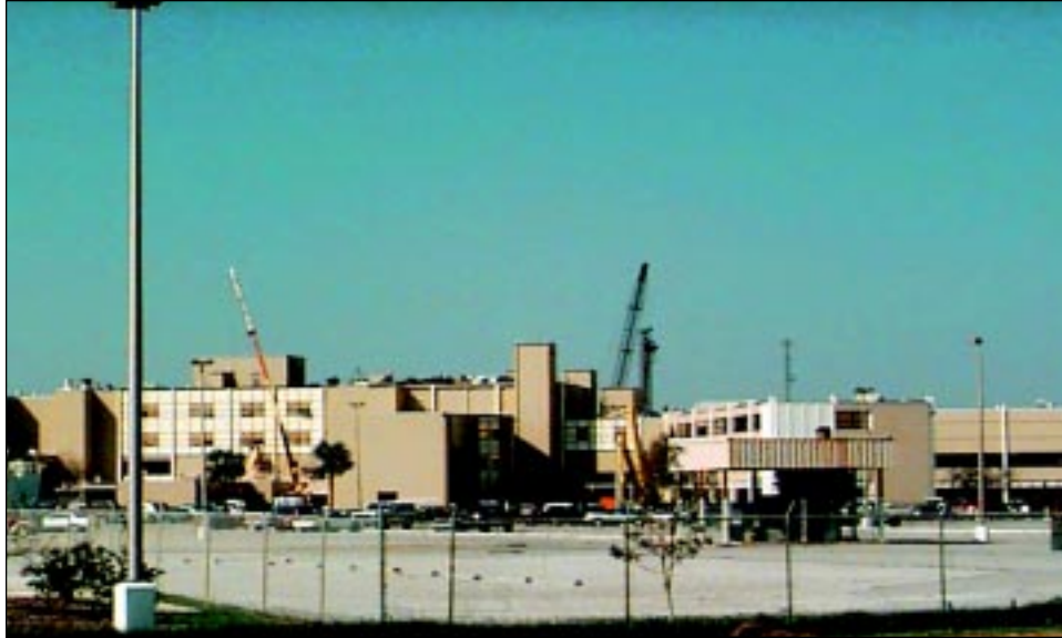
FIGURE 6-18 Singing River Hospital, where emergency roof repairs are underway.
