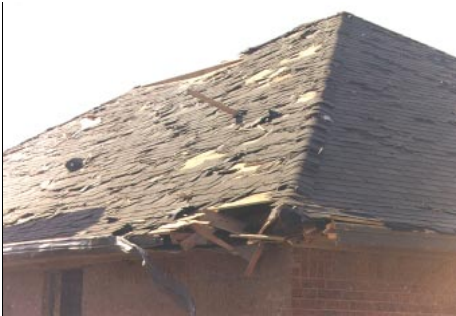
FIGURE 4-14: Asphalt shingles covering roof of residential home.
