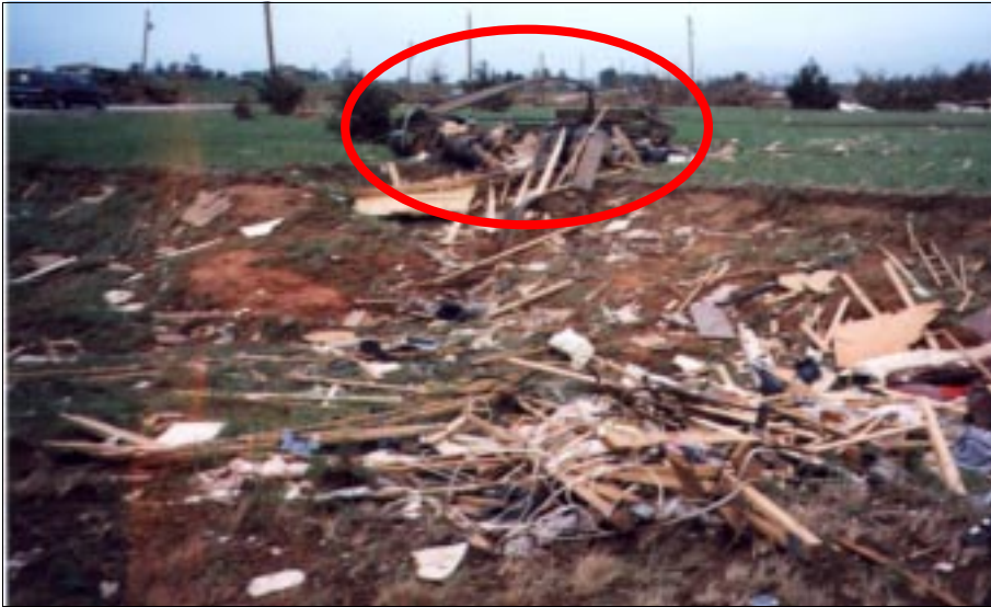
FIGURE 4-48: This 14-ft x 60-ft manufactured home chassis in the background of this picture moved about 200 yards from its original anchoring site in Figure 4-49, Bridge Creek, Oklahoma.
