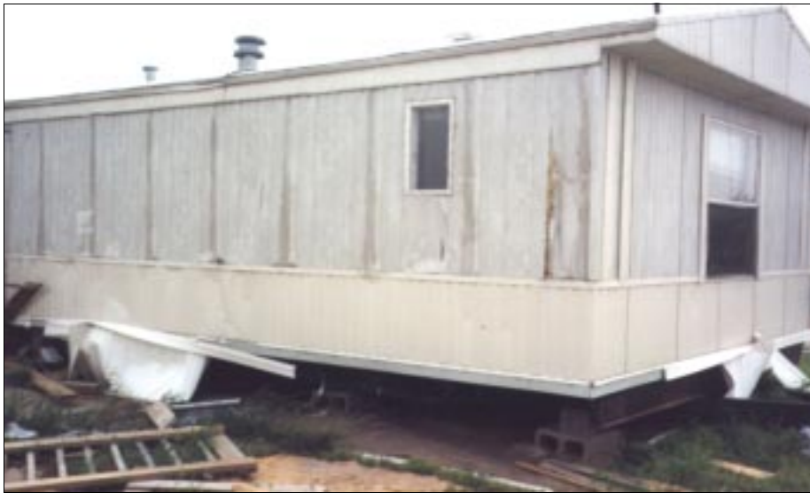
FIGURE 4-58: This manufactured home laterally shifted from wind force generated along the periphery of a violent tornado, Haysville, Kansas.
