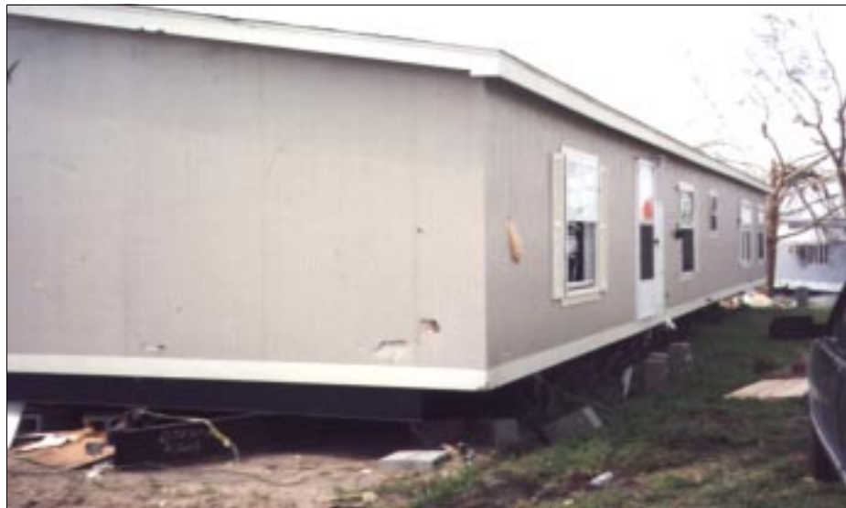
FIGURE 4-61: Manufactured home laterally shifted from wind force generated along the periphery of a violent tornado, Wichita, Kansas.
