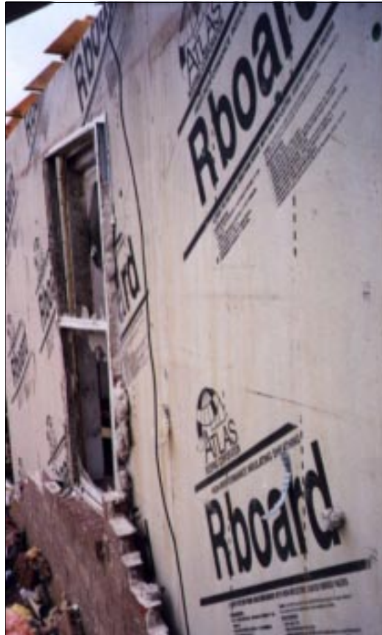
FIGURE 4-34: Inadequate bonding of mortar to galvanized brick ties, Bridge Creek, Oklahoma.
