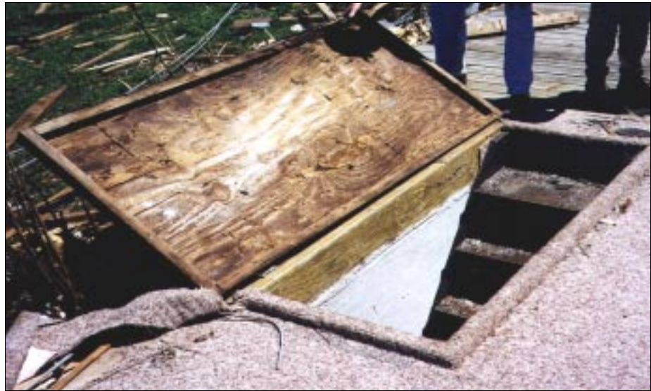
FIGURE 3-29: Underground residential shelter, viewing door and stairway leading down to shelter. This shelter was located outside a residence.
