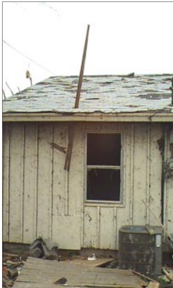
FIGURE 3-16: A missile vertically striking the roof of a home in Mid West City, Oklahoma. It fell nearly vertical illustrating the importance of a strong cover over the top of a tornado shelter to protect against free-falling debris.
