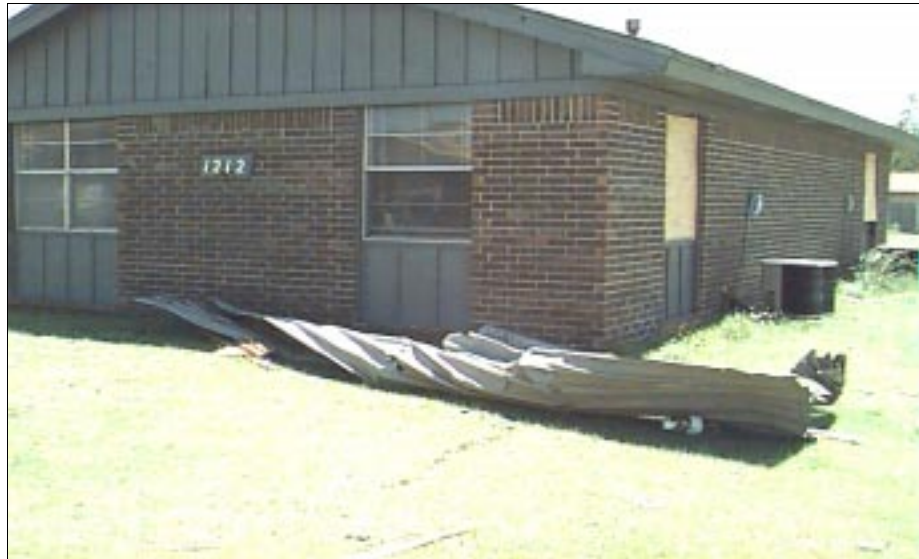
FIGURE 3-21: This piece of steel deck landed at the periphery of a violent tornado damage area in Moore, Oklahoma. The building it likely came off of was a few hundred feet away.
