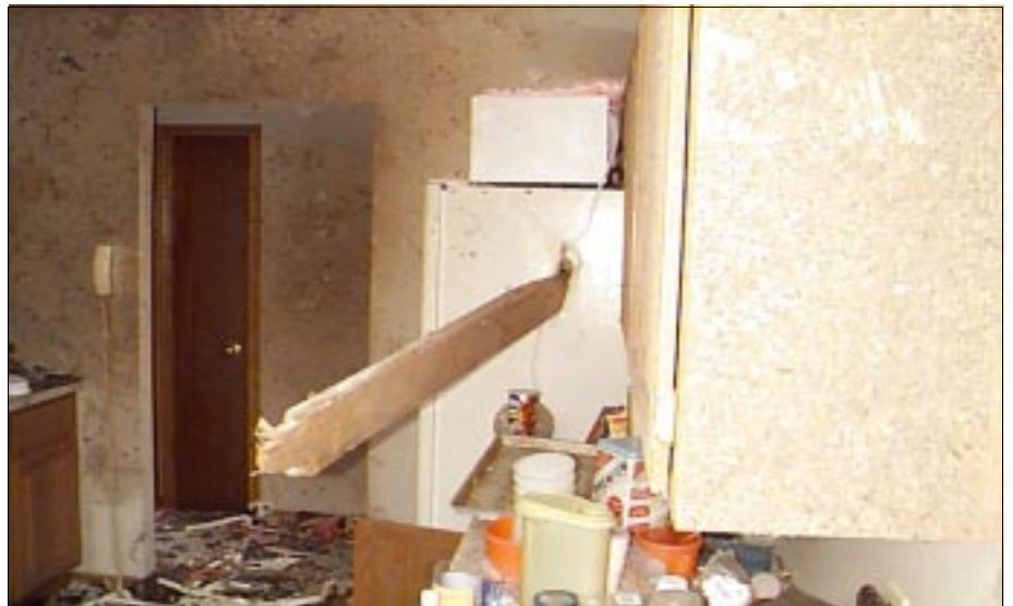
FIGURE 3-18: A 2-in by 6-in board missile penetrating a refrigerator located inside a home in Country Place subdivision outside Oklahoma City, Oklahoma.
