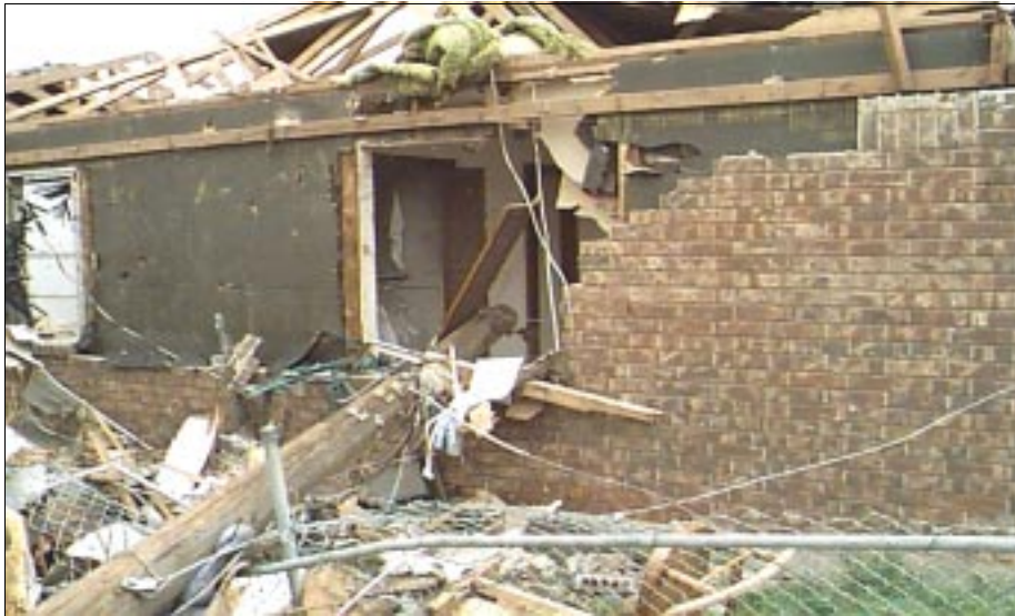
FIGURE 3-19: This power pole penetrated a window and extended several feet into the house after traveling approximately 40 feet from its original location. This home was located in Moore, Oklahoma, along the track of a violent tornado.
