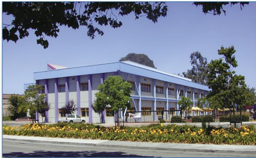
Figure 1-10 Private high school, Palo Alto, CA, located in a remodeled industrial building. Note the exterior cross bracing; the building required extensive retrofitting to meet school seismic requirements.
