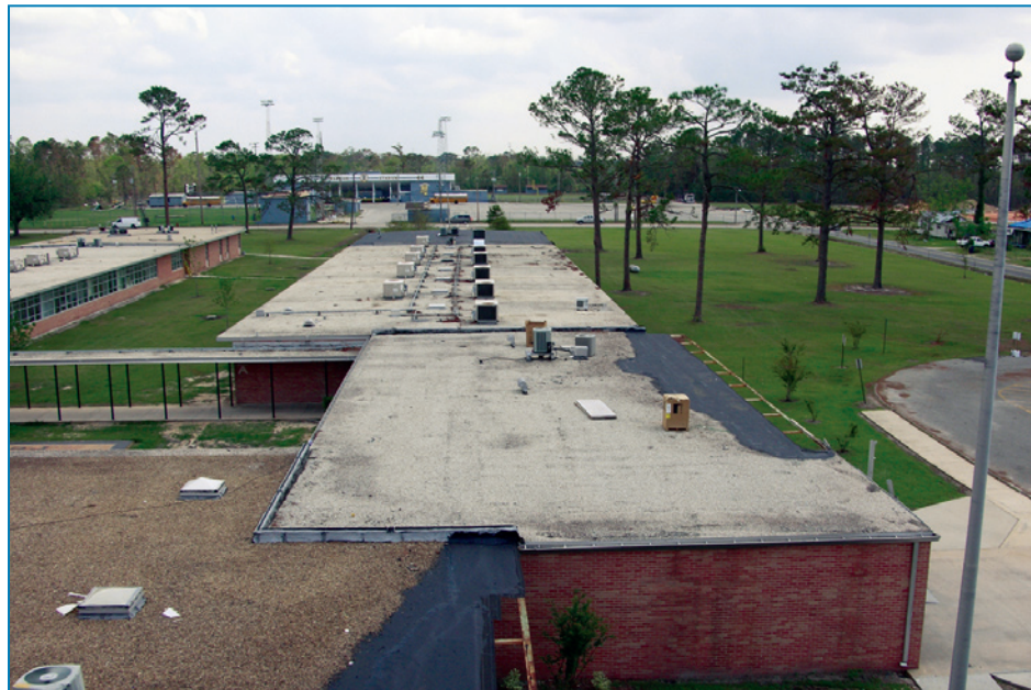
Figure 4-112: The cementitious wood-fiber deck panels detached from the joists along the overhangs and caused the built-up membranes to lift and peel. Hurricane Katrina (Mississippi, 2005)
