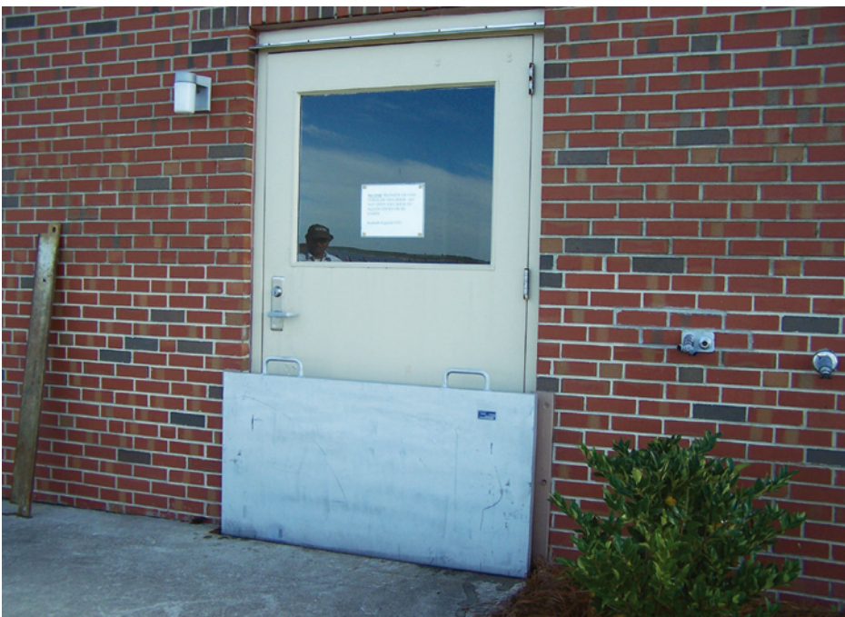
Figure 3-46: Most of the panels can be installed by hand. Note the protective metal strip leaning against the building on the left; normally this strip covers the horizontal channel into which the panel is inserted.
