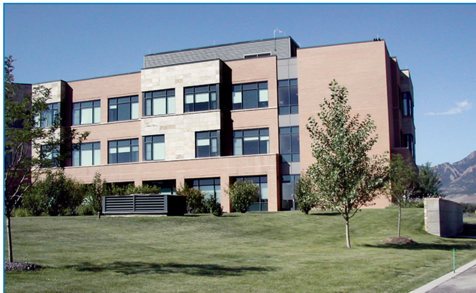
Figure 3-35: The upper floors provide patient care. The top of the retaining wall (on right) and the air handler (left of center) are approximately one-foot above the 500-year flood elevation.
