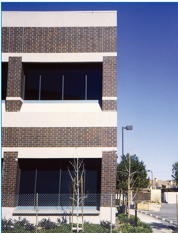
Figure 2-17: A steel frame building with a post-earthquake "lean" to the right, seen particularly at the first floor. Severe damage was found in its beam-column joints and it was later demolished.
