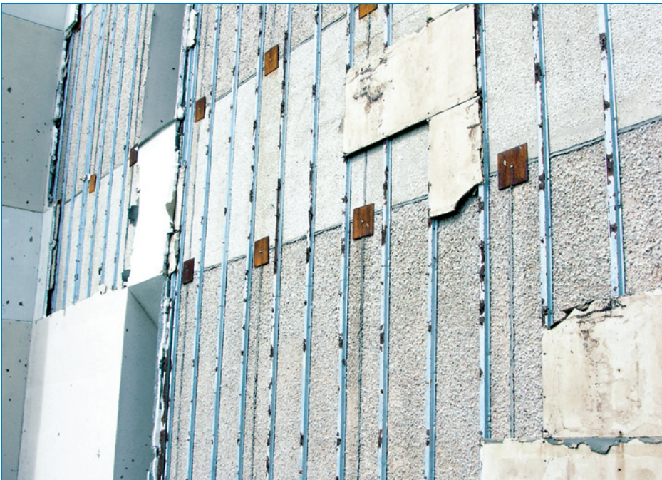
Figure 4-23: Close-up of the damaged EIFS at the hospital. In this area most of the insulation and gypsum board was blown from the steel furring channels.
