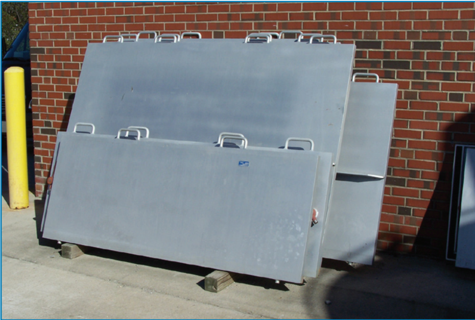
Figure 3-45: Large floodproofing panels are stored at the hospital, ready for installation when coastal flooding is predicted.
