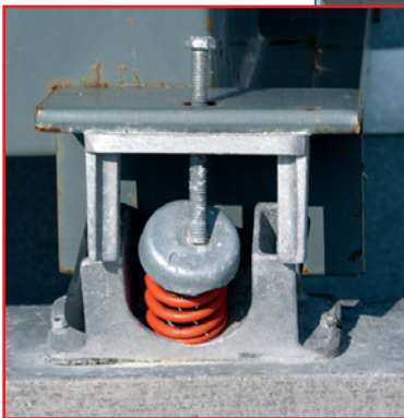
Figure 4-92: Failure of vibration isolators that provided lateral resistance but no uplift resistance caused equipment damage. A damaged vibration isolator is shown in the inset. Hurricane Katrina (Mississippi, 2005)
