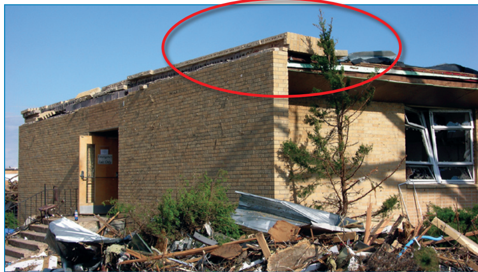
Figure 4-139: Collapsed unreinforced masonry parapet. Note the broken windows.
