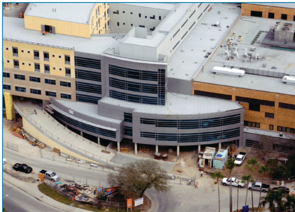
Figure 3-40: Tampa General Hospital solved the problem of access to the new elevated Emergency Department by designing a vehicle ramp. Visitors and ambulatory patients take elevators from the ground floor.
