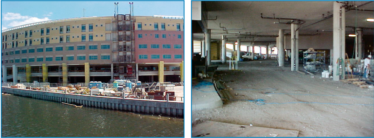
Figure 3-29: Tampa General Hospital had its new Emergency Department wing designed to be elevated on columns, well above hurricane storm surge flooding elevations.
