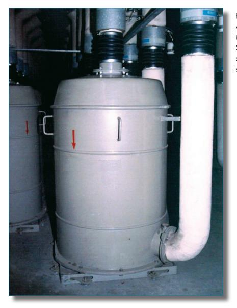
Figure 3-4 A canister-type filter unit is often used for Class 1 Safe Rooms to maximize storage life of the filters. SOURCE: BATTELLE
