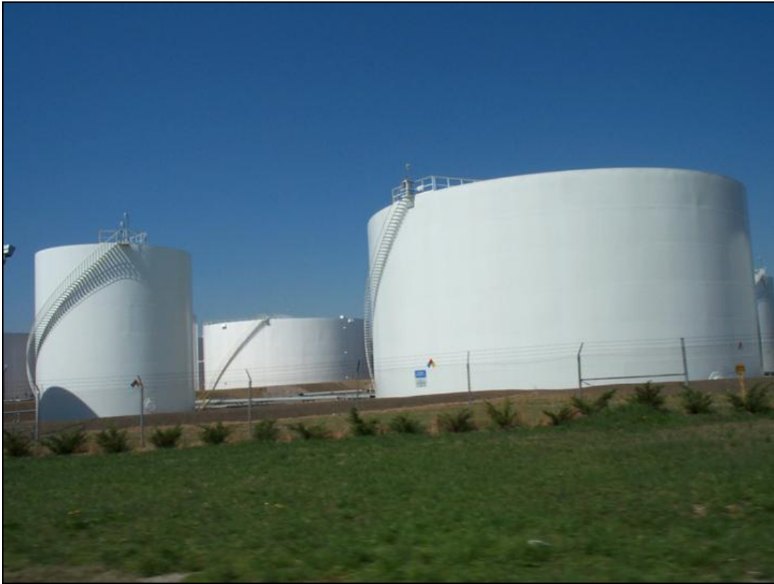
Figure 35. Shellexxico Tank Farm
