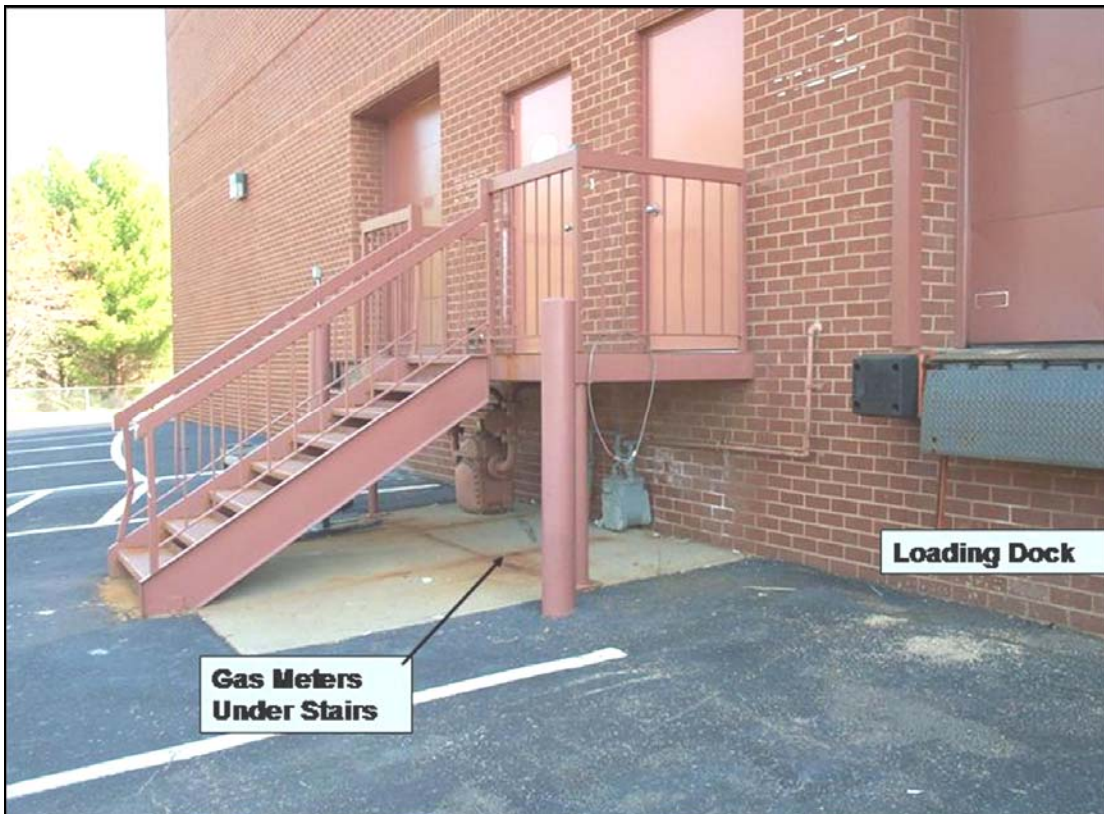
Figure 17. Loading Dock Area
