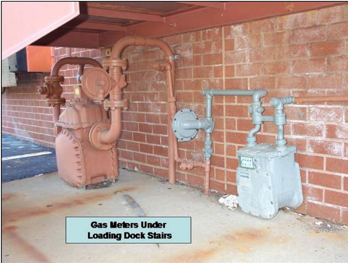
Figure 18. Gas Meters Under Loading Dock Stairs
