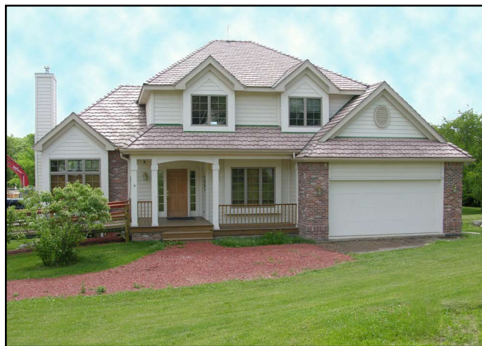
The Research Demonstration House, built on FPL grounds, is being used to monitor moisture intrusion and promote proper building practices.
